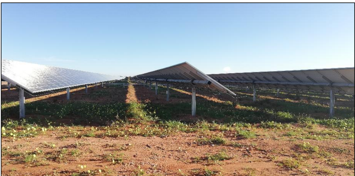
Figure 4: Photographic Example of Single portrait tracker PV (Photo – Cape EAPrac, 2019)
