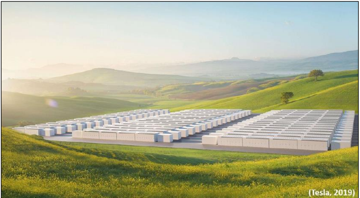
Figure 6. Artist's impression of a Tesla Battery Energy Storage System (BESS) in landscape.
