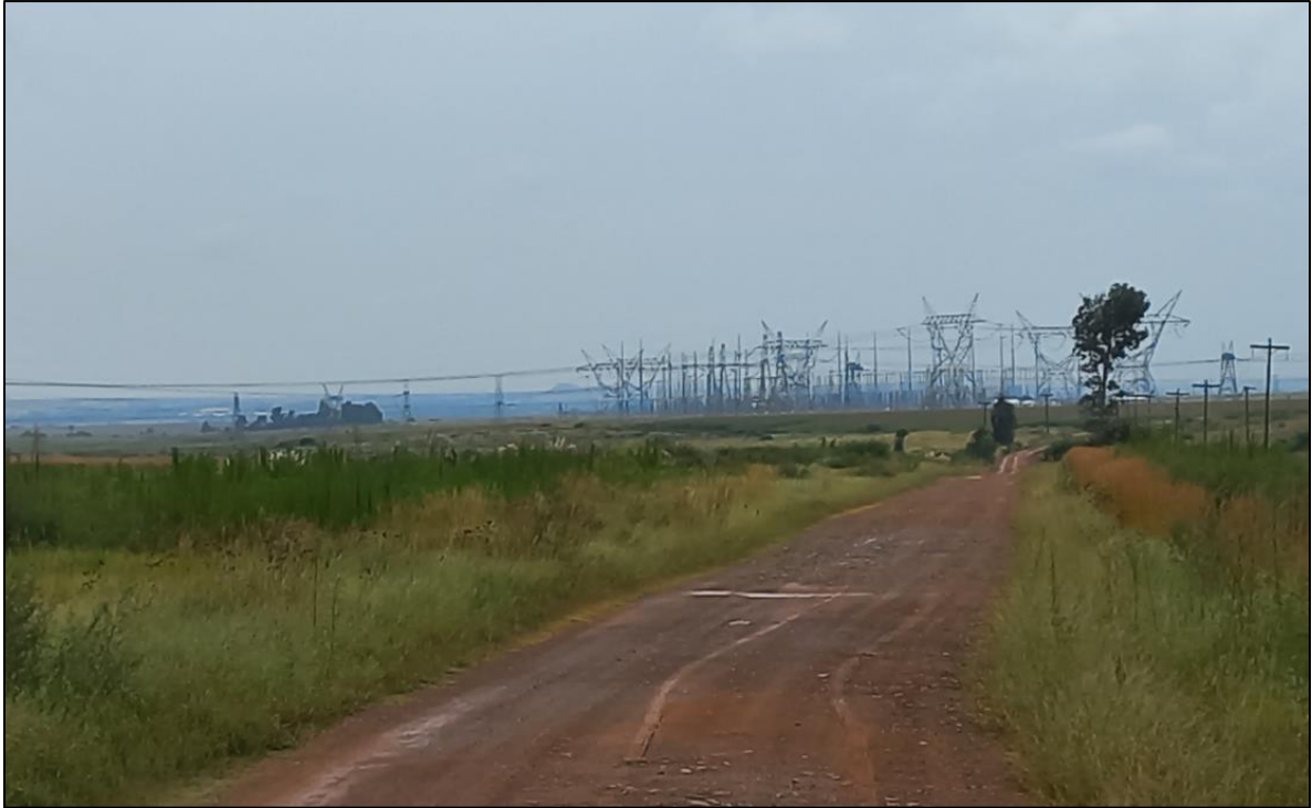
Figure 14: Photograph of the Eskom Mercury Substation.
