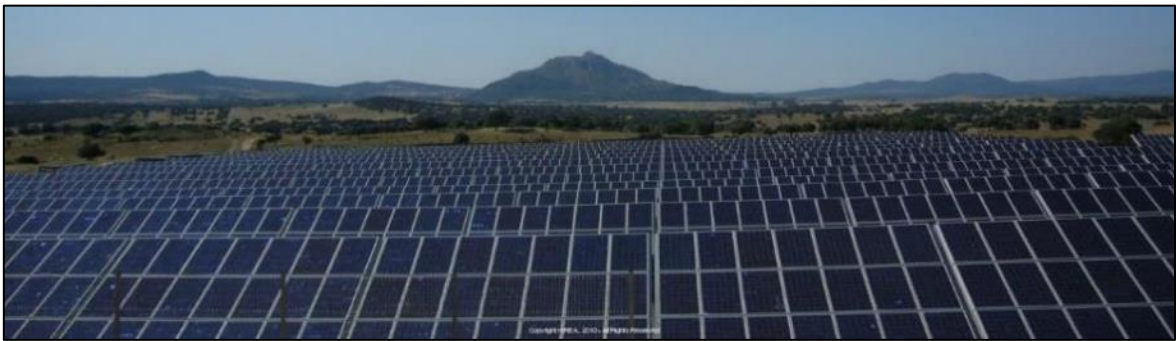
Figure 3: Photographic Example of Rows of PV panels (www.hawaiirenewableenergy.org/Villamesias2, n.d.)
