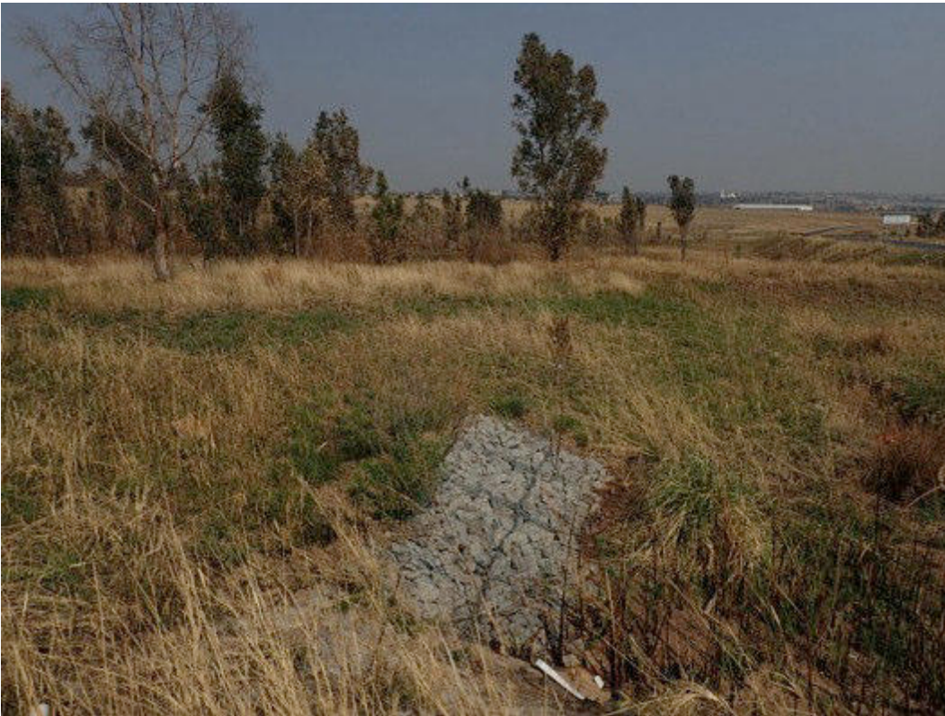
Figure 44 Storm water outlet under the access road to the Waterfall Cemetery
