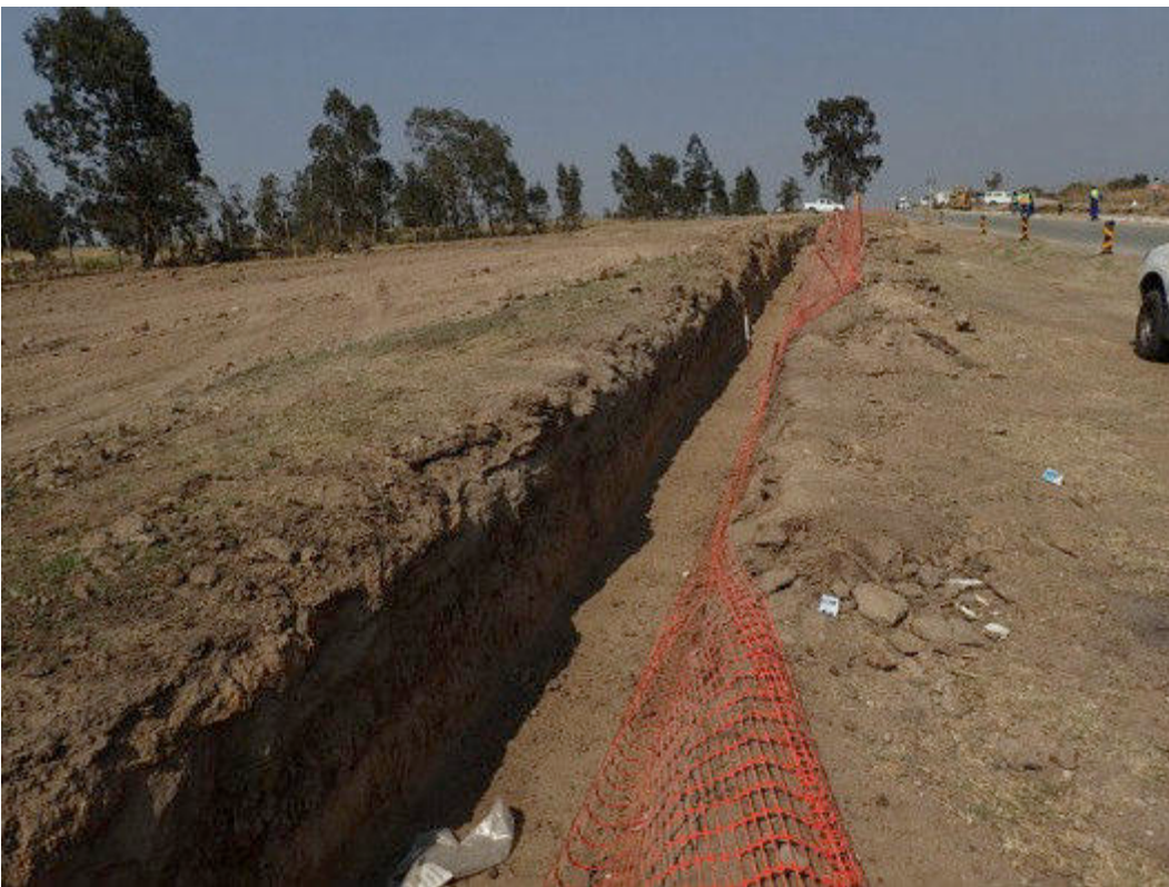
Figure 35 Current road works and trenching on Site 2
