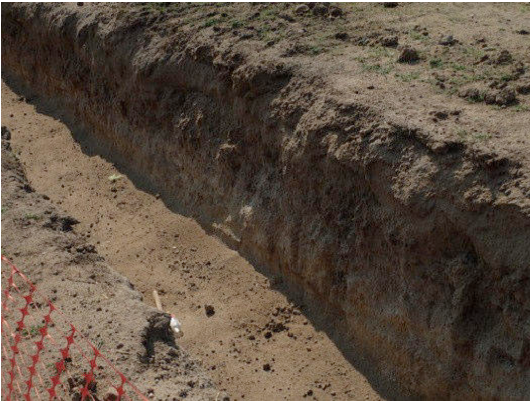
Figure 34 Current road works and trenching on Site 2
