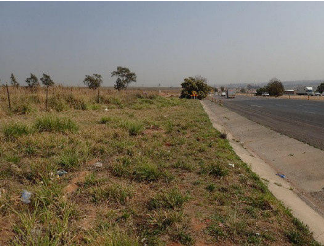
Figure 32 View of Site 2 towards the north west with Allandale Road and its storm water infrastructure evident
