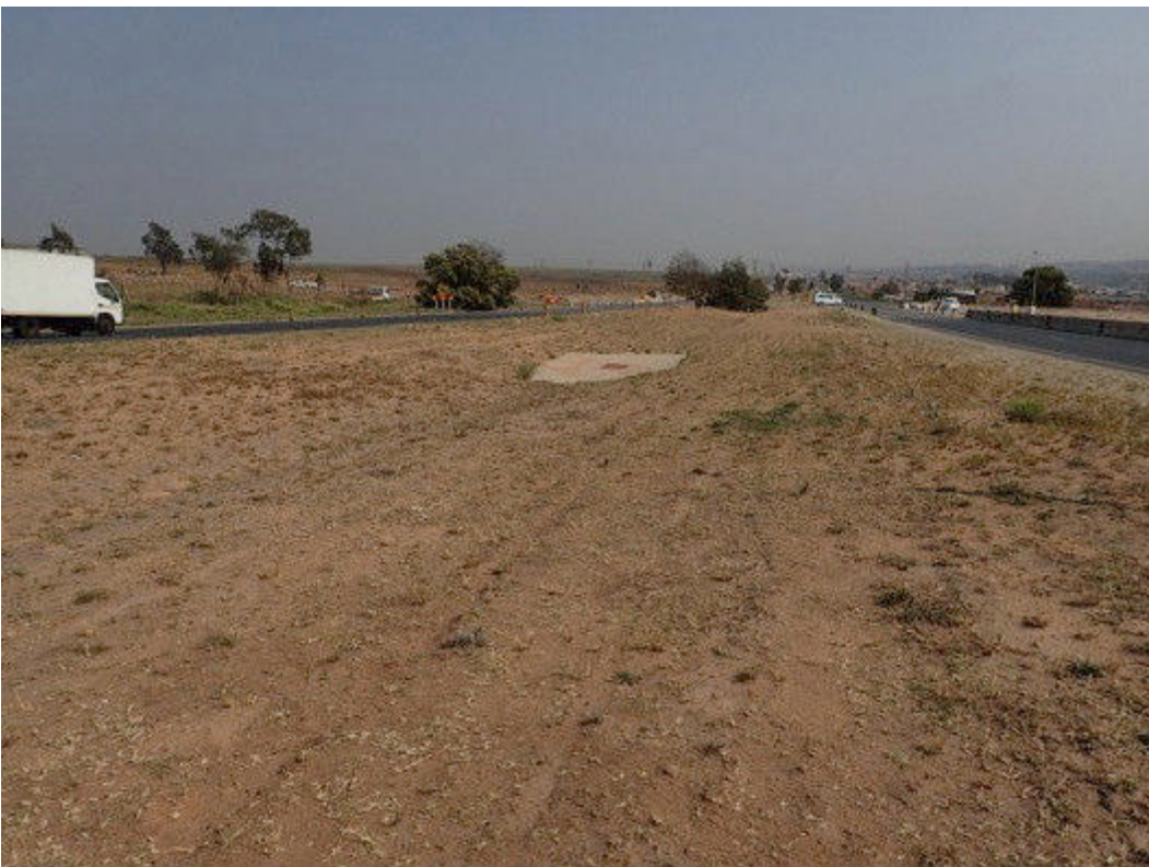
Figure 29 View of Site 2 towards the northwest with a storm water inlet between the two lanes
