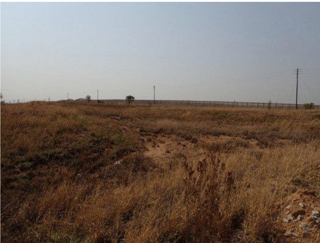
Figure 47 Storm water channel (unlined) running parallel to Alsatian Road above the access road to the Waterfall Cemetery
