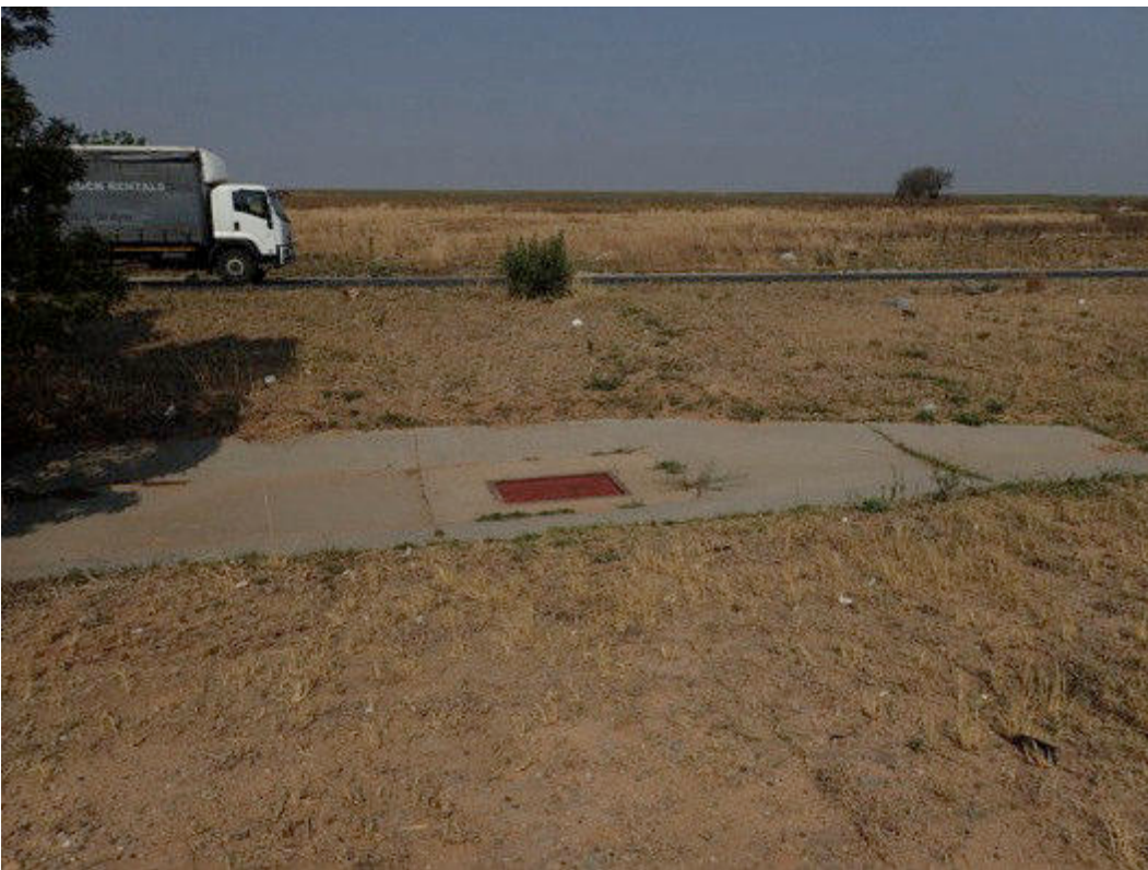
Figure 42 Storm water inlet on Allandale Road on Site 2 between the roadways
