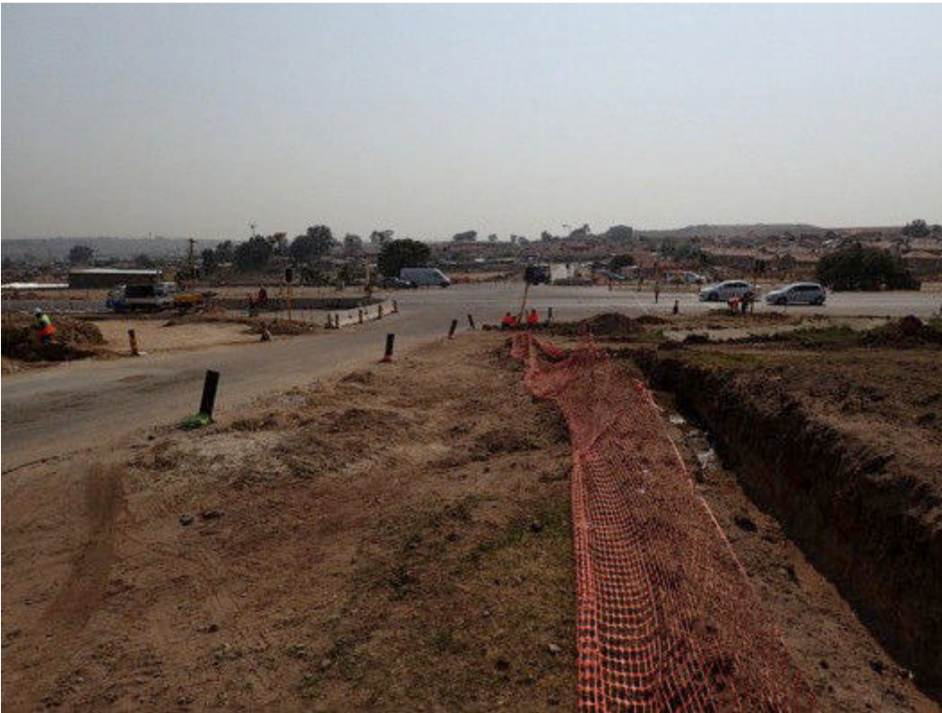
Figure 36 Current road works and trenching on Site 2
