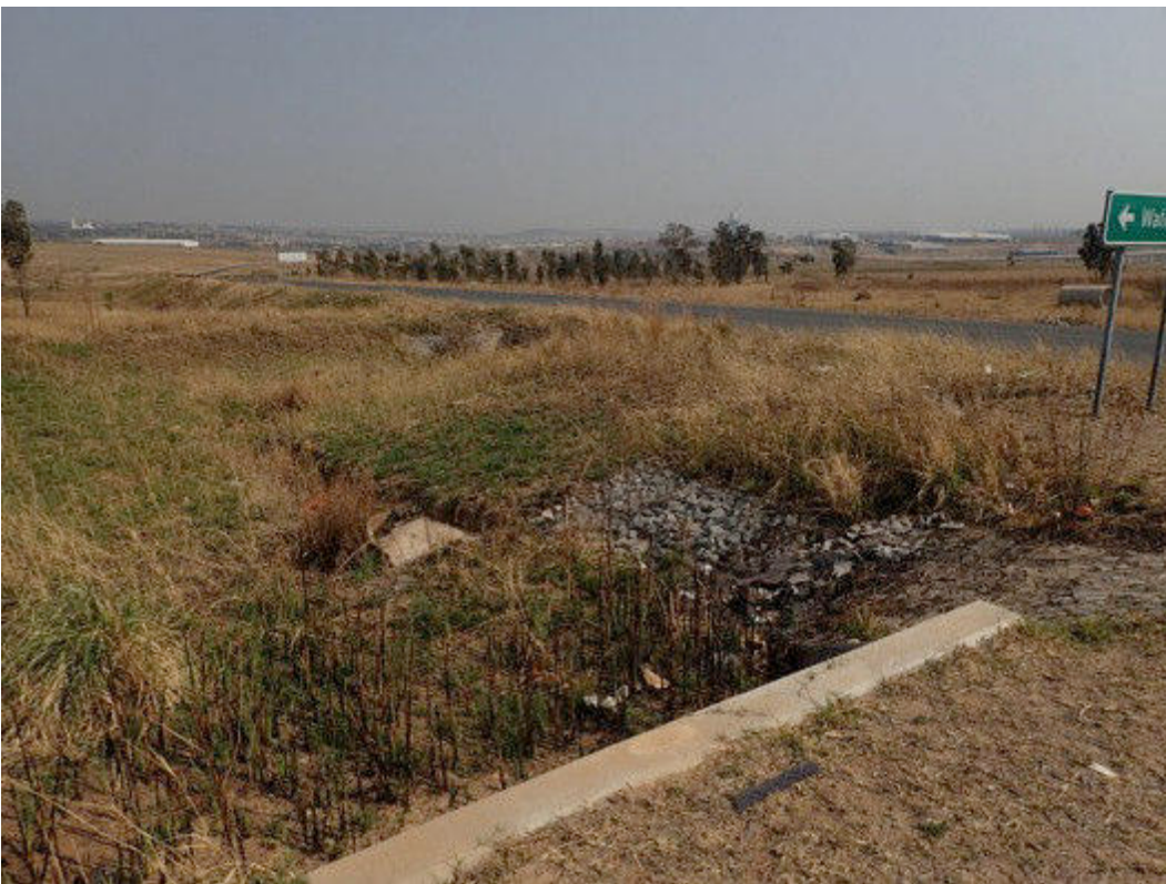
Figure 45 Storm water outlet under the access road to the Waterfall Cemetery
