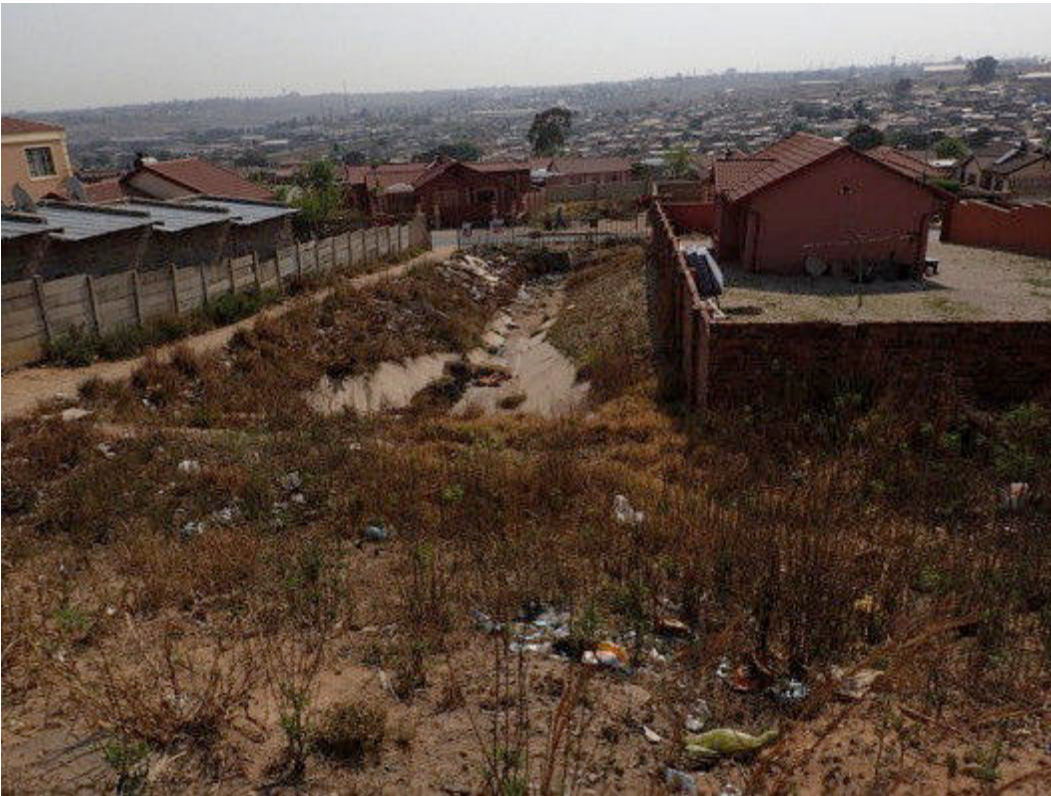
Figure 43 Storm water outlet on Site 2 towards the north of Allandale Road
