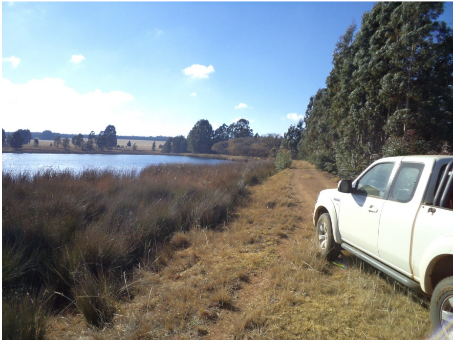
Photograph 2 Right Bank Crest
