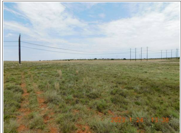
Photograph 8: Tributary and grasslands crossed by overhead powerlines
