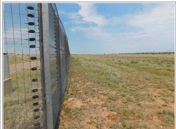
Photograph 10: Fencing around solar panels; electrified component facing inwards toward discrete infrastructure
