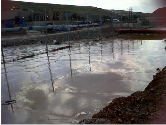
Overflow of toxic and radioactive water from Pump Station No 2
