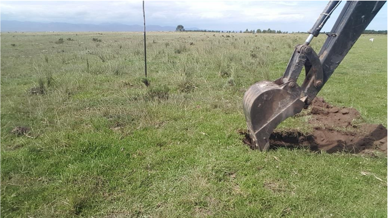
Figure 6. Photograph showing excavation of test pits in typical site conditions.
