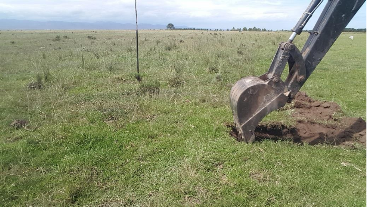
Figure 6. Photograph showing excavation of test pits in typical site conditions.
