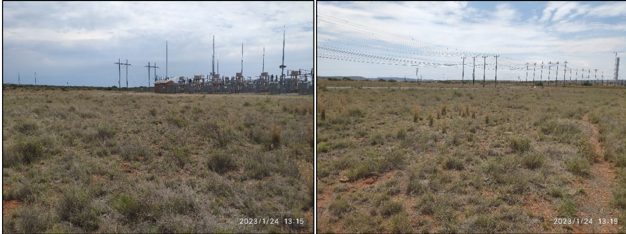
Photo plate 6: Open grassy vegetation around the substation
