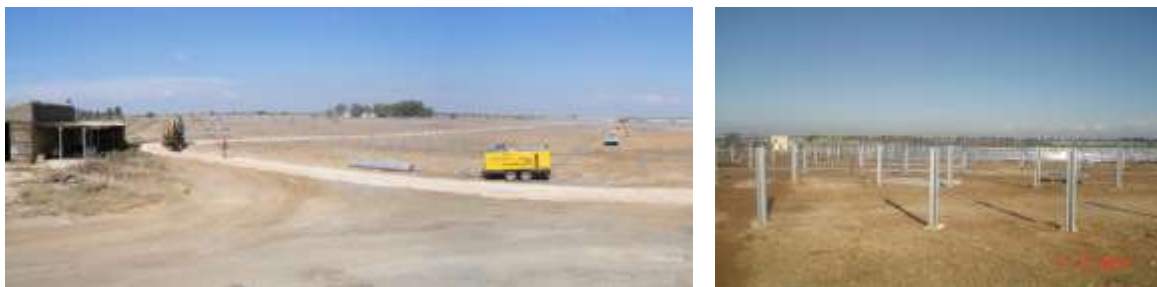
Figure 18: Illustration of a typical site after preparation
