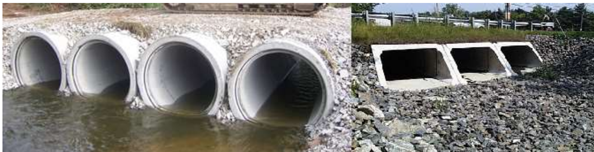
Figure 14: Installed concrete pipes and culverts
