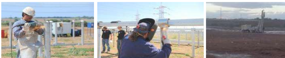
Figure 19: On-site construction of the PV arrays
