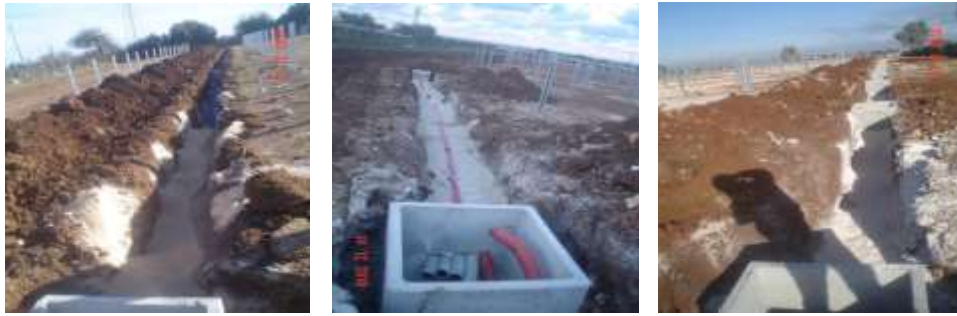
Figure 9: Typical cable trenches.
