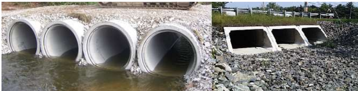
Figure 14: Installed concrete pipes and culverts (illustration)
