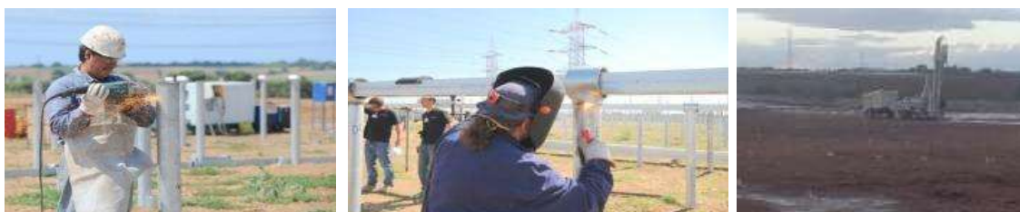
Figure 19: On-site construction of the PV arrays
