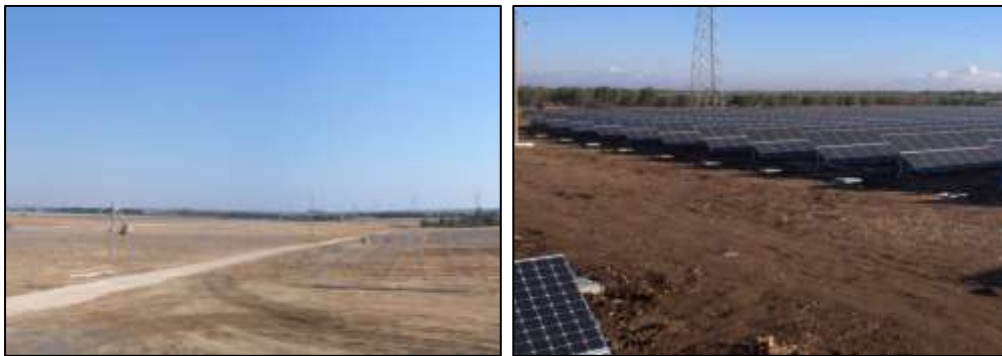
Figure 6: Typical internal road example
