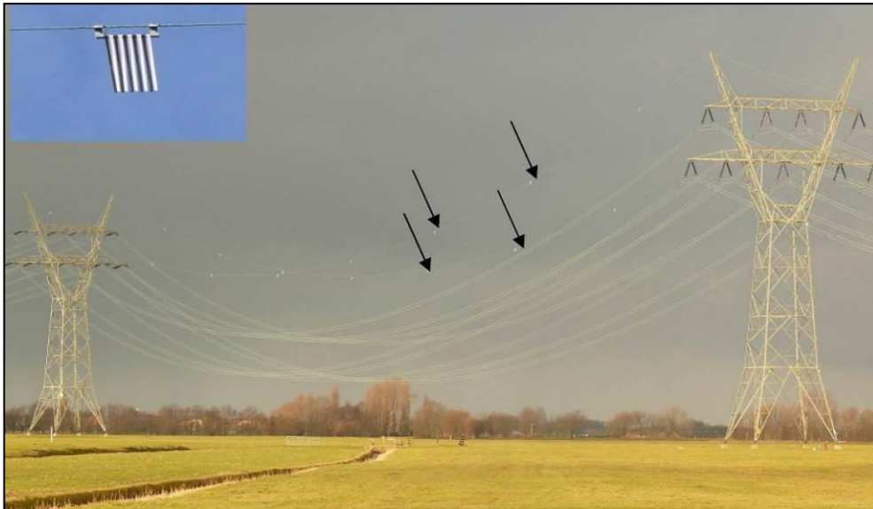
Photograph 8. High tension (150 kV) power line in the Netherlands with bird flappers (see arrows) placed at regular intervals in both ground wires as bird flight diverters, see also Box 1 (Photo: Bureau Waardenburg)
