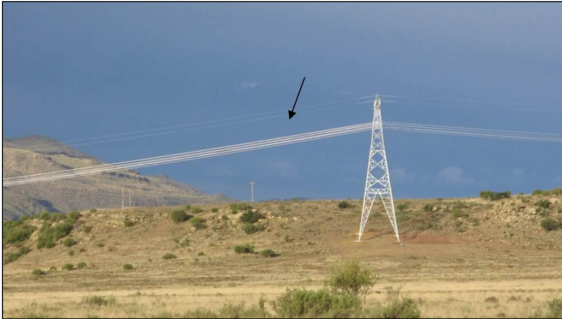
Photograph 9. A 400 kV line, with all conductor wires in the same horizontal plane (Photo: EWT-WEF)
