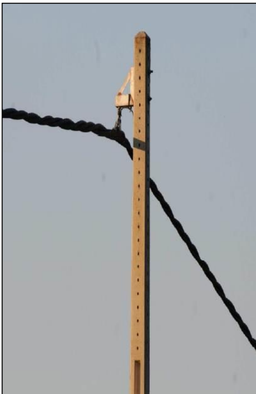
Photograph 5. Completely insulated medium tension cable hanging from concrete pole without need of insulators (source: Haas, 2011)
