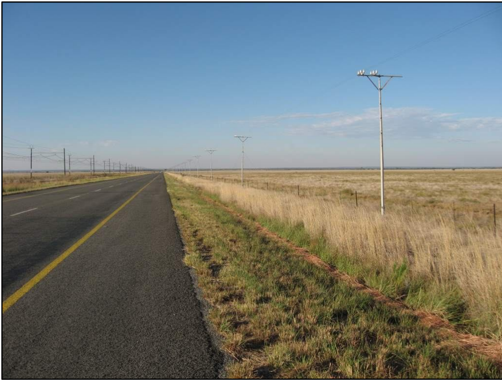
Figure 3 – View of to the N12 towards Kimberley (Study area on the right)
