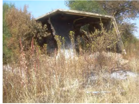
Old drive-in entrance building
