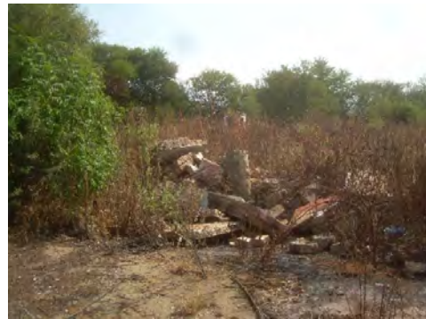
Rubble on site
