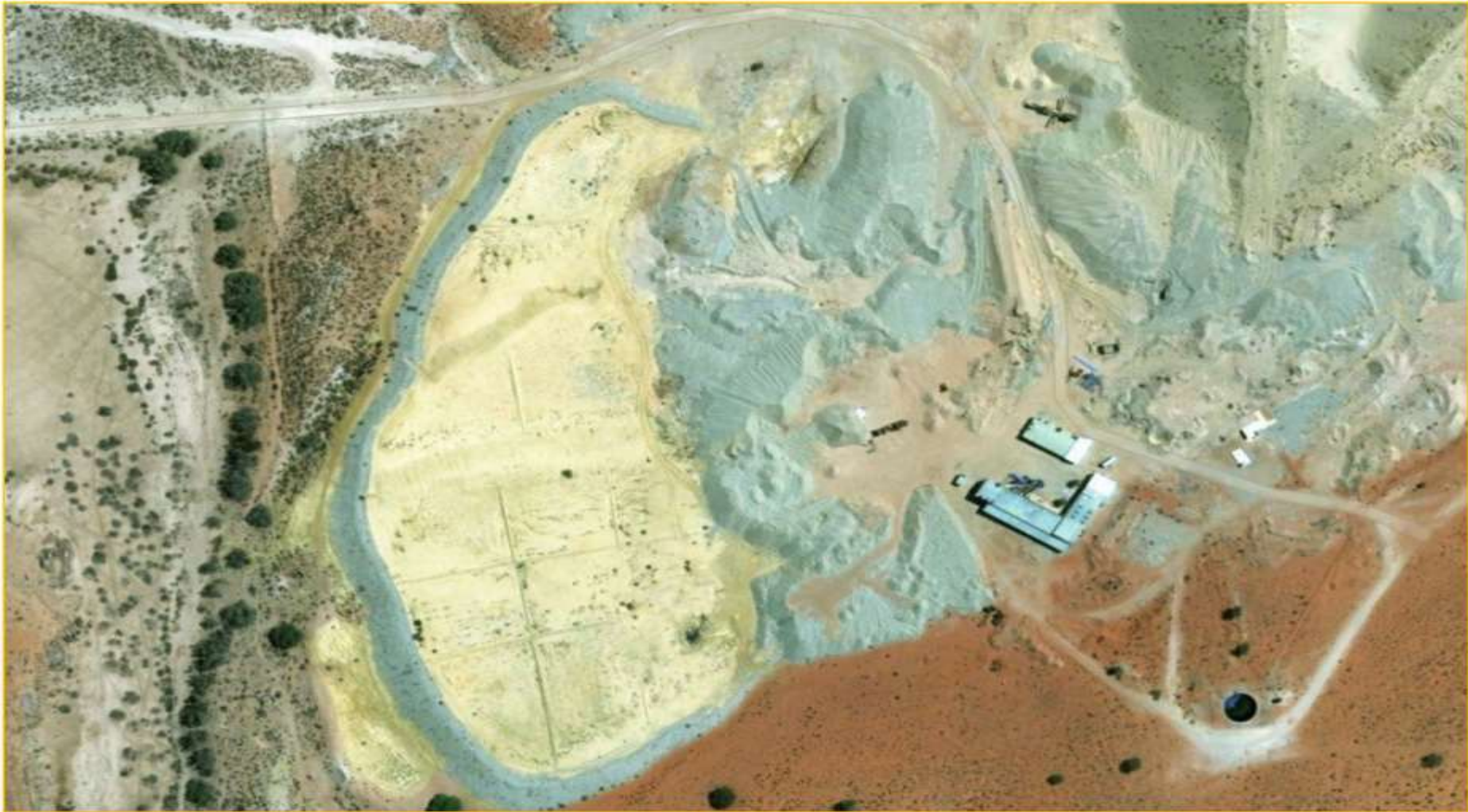
Figure 2. A plan indicating the overall location and extent of listed activities and main infrastructure
