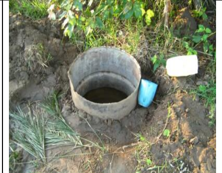
Photo 2.7 Informal water abstraction well in river bed (Hlazane River at Gwalabanda).
