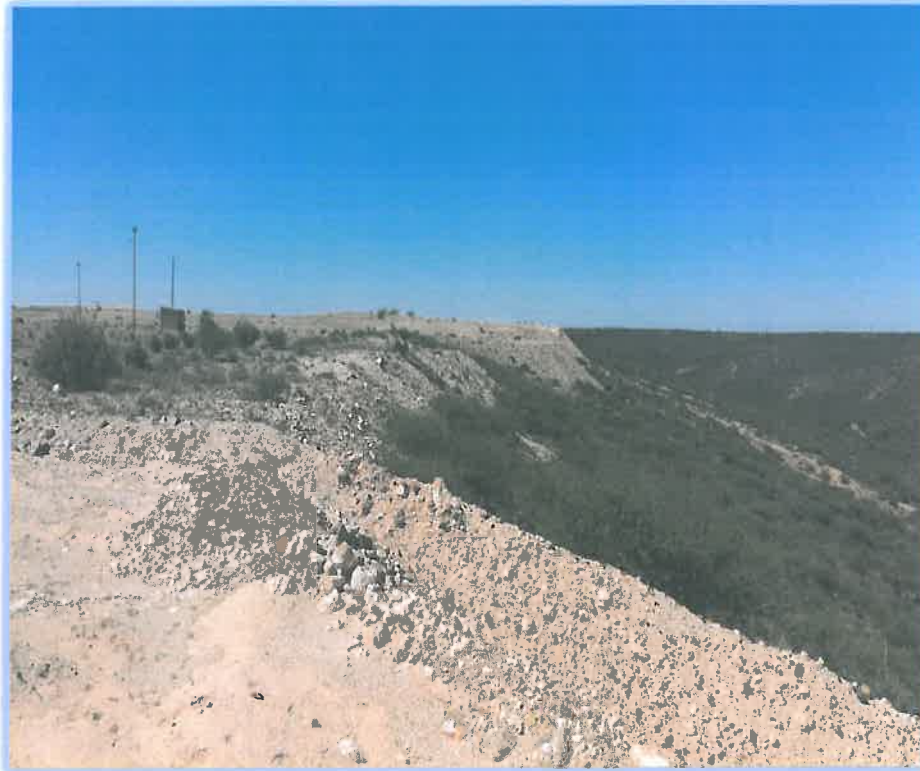
Plate 5: The brick toilet structure and lighting poles on the existing disturbed areas
