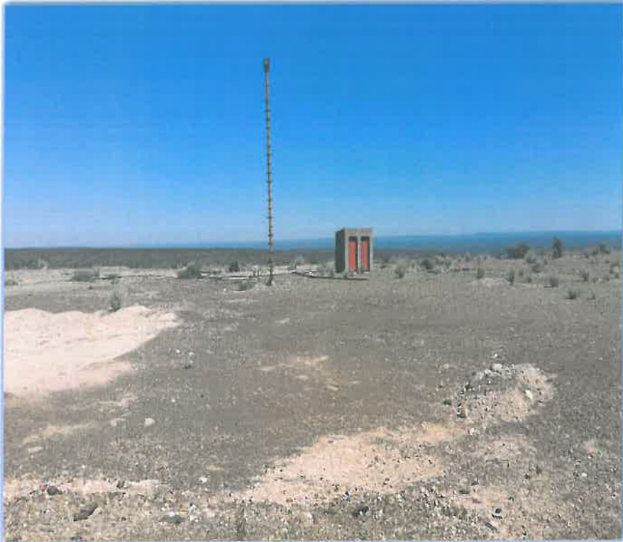
Plate 3: Existing toilet brick building and lighting pole
