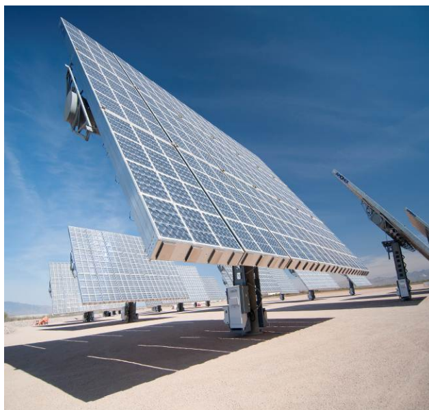
Figure 2.4: The support structures elevate the panels and allow for dual axis tracking of the sun for increased efficiency (Source: AmonixTM)
