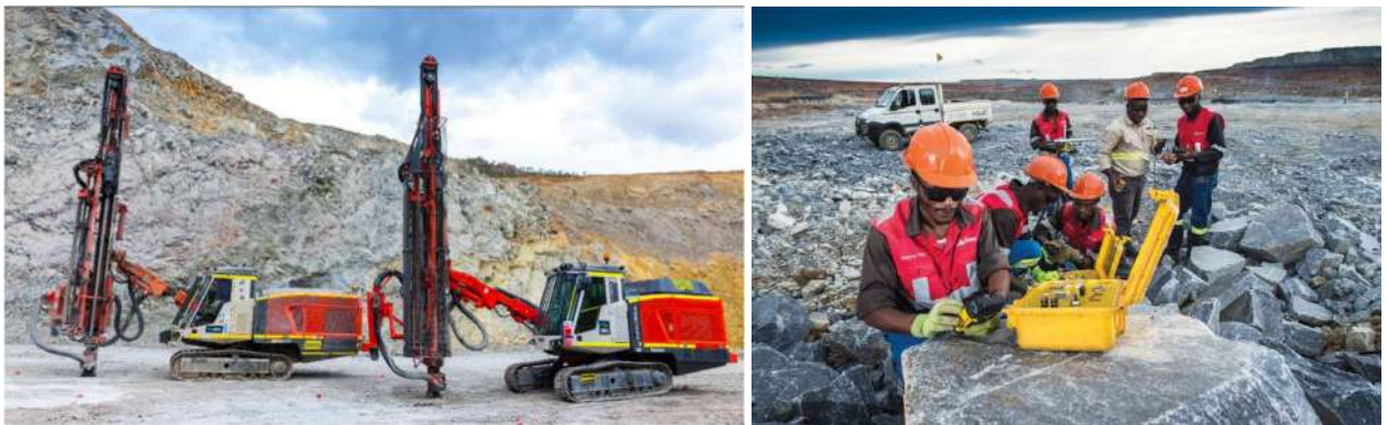
Figure 79: Typical example of blasting operation.
