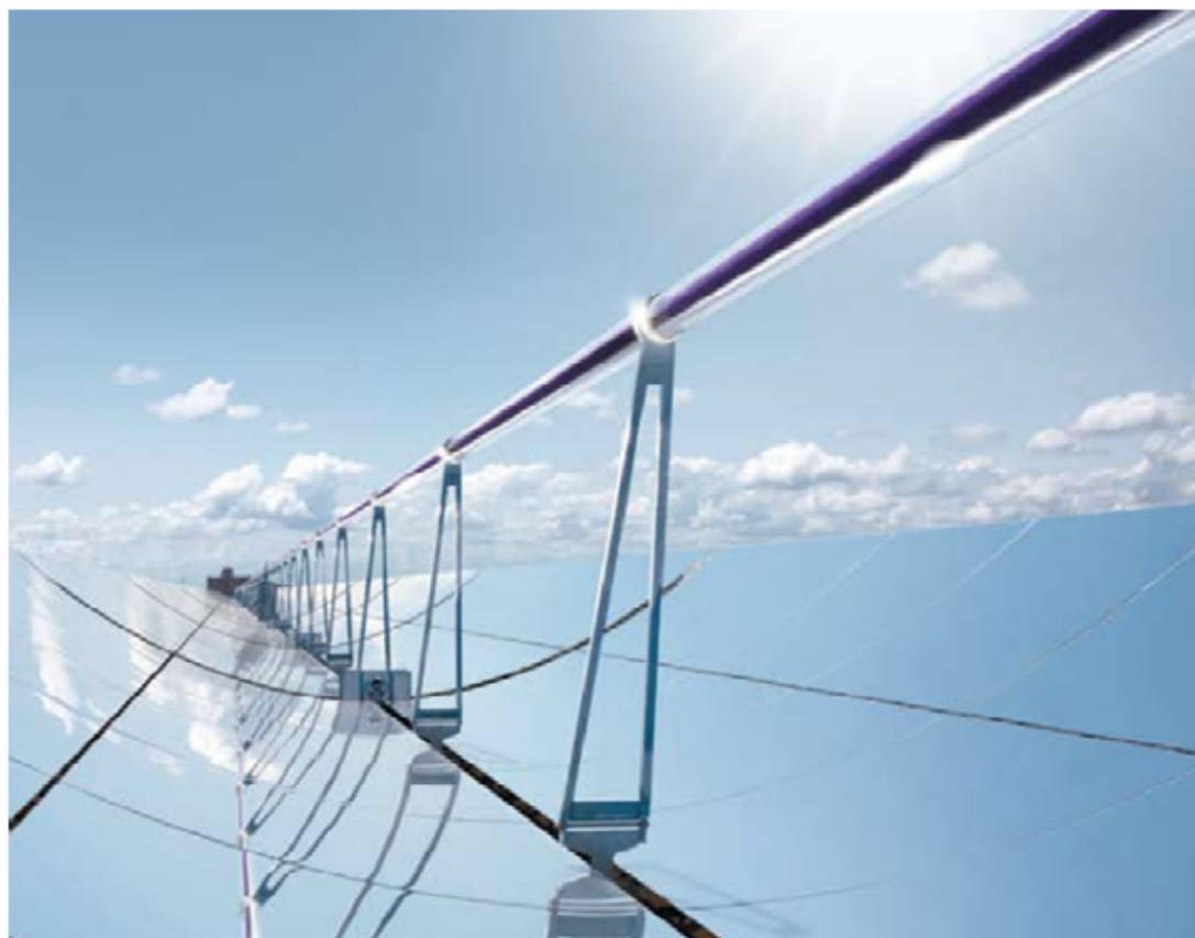
Figure 2.1: The top photograph illustrates the pipes conveying the heat transfer fluid and the bottom photograph illustrates the parabolic troughs together with the receiver tube
