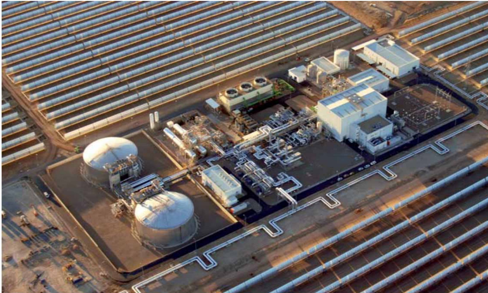
Figure 2.5: Aerial view of a concentrating solar plant utilising parabolic trough technology with storage
