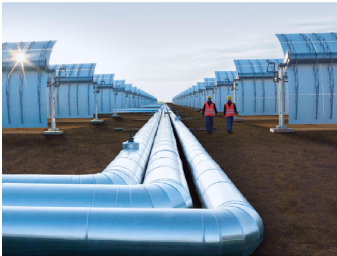
Figure 2.2: The pipes lain between the troughs convey the heat transfer fluid (Source: Siemens AG)
