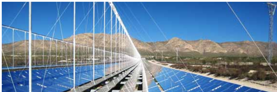
Figure 2.5: Linear Fresnel technology (Source: Novatec)
