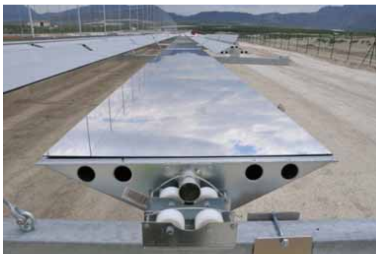
Figure 2.6: Primary reflector (Source: Novatec)
