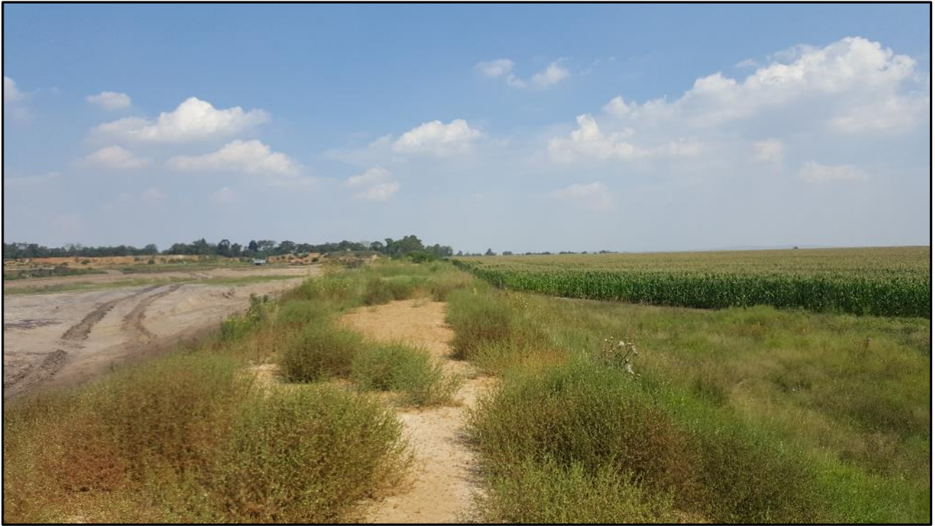
Figure 13: View of the berm on the border of the existing Vlakfontein quarry and the study area to the south-east
