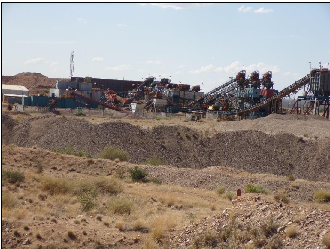
Figure 9: Evidence of previous mining infrastructure still on site
