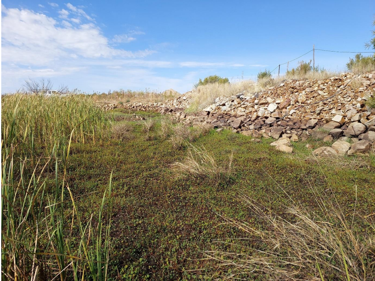
Figure 24: Infilled road and berms disturbing the western part of UVB1 middle.
