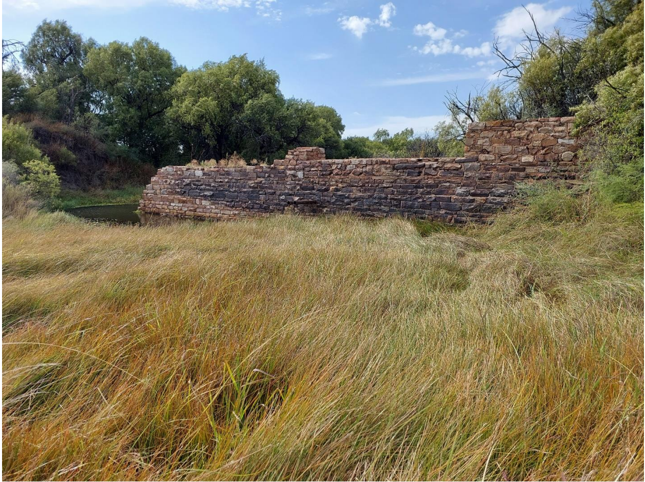
Figure 23: Old dam wall, likely the cause of the deep pool of water within the middle of the UVB1 upper section & riparian zone.
