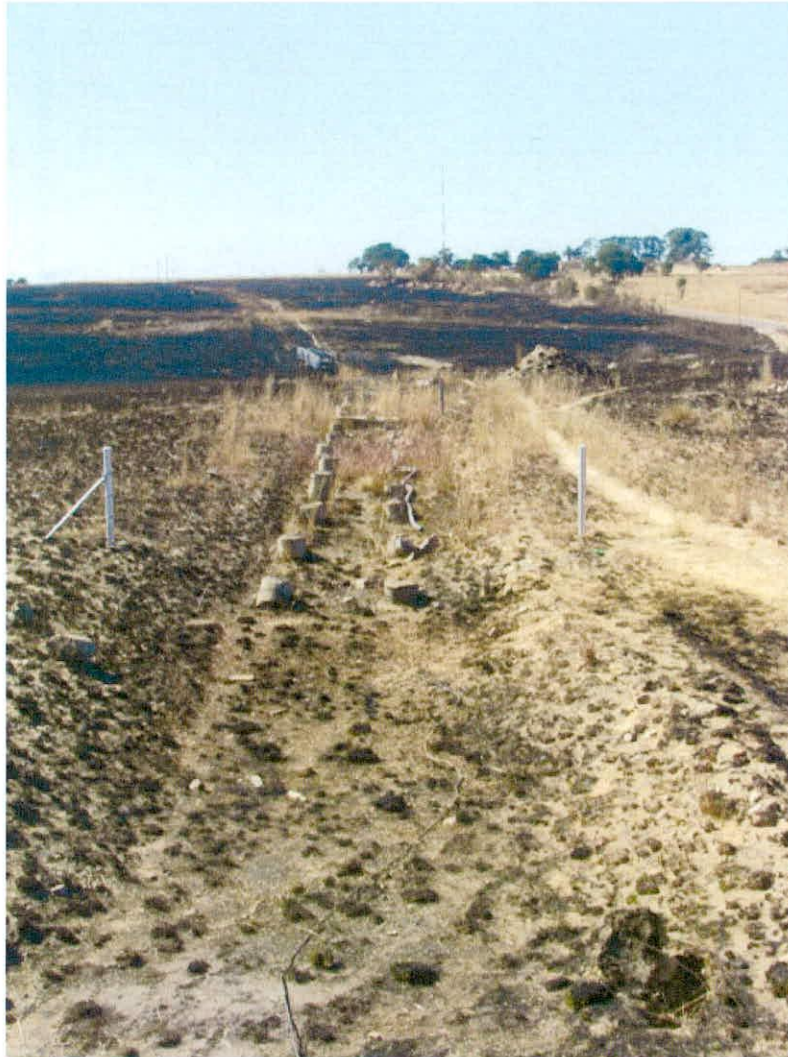
Figure 5 A view along the route of the conveyor. Note the remains of the former conveyor.
