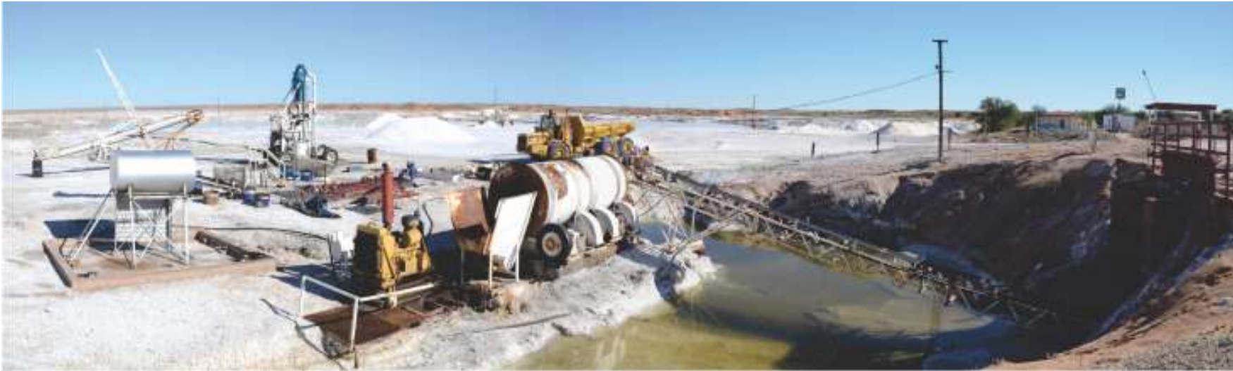
Photo 7: Overview of the washing / processing plant at the site.
