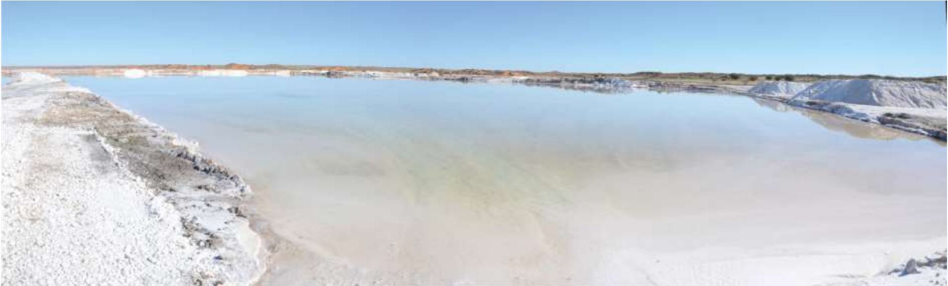
Photo 12: Typical Evaporation pond. Note the "dam" wall at less than 1.5m in height and the shallow nature of these evaporation ponds
