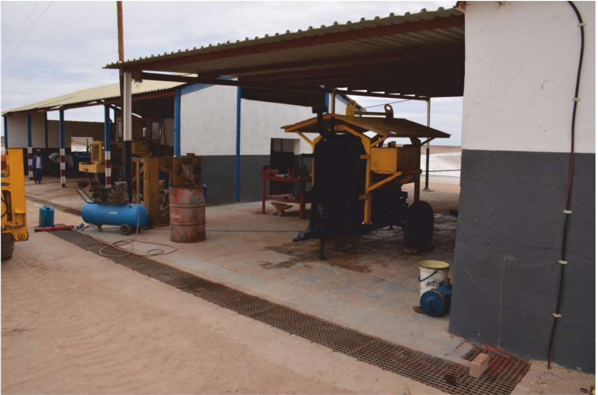
Photo 11: Workshop showing concrete working apron and drain leading to oil trap.
