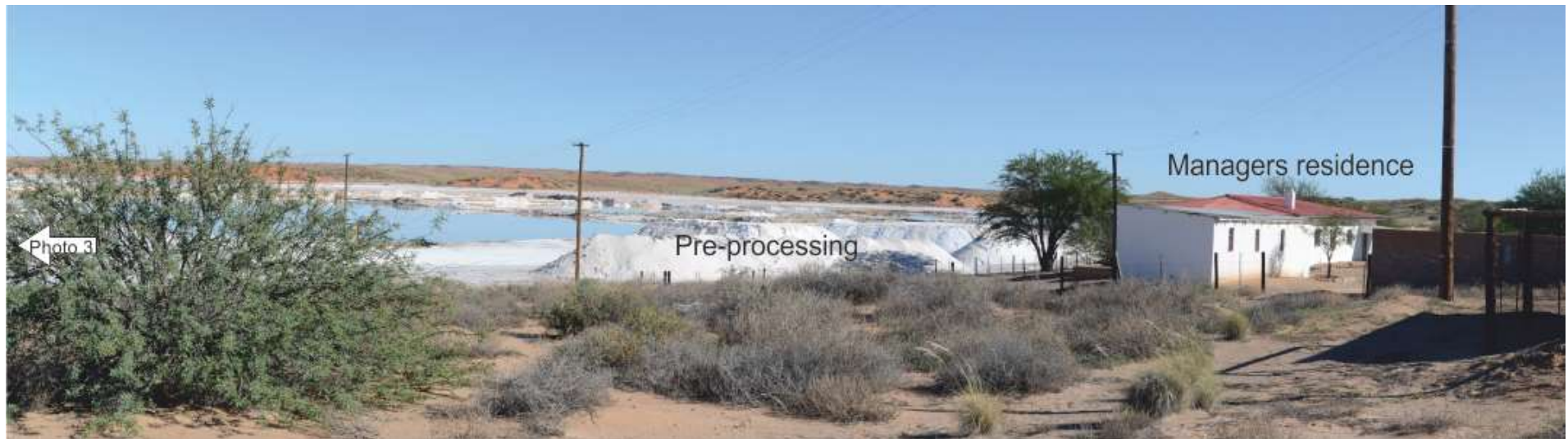
Photo 4: Looking north and west from Generator house showing overall view of operations
