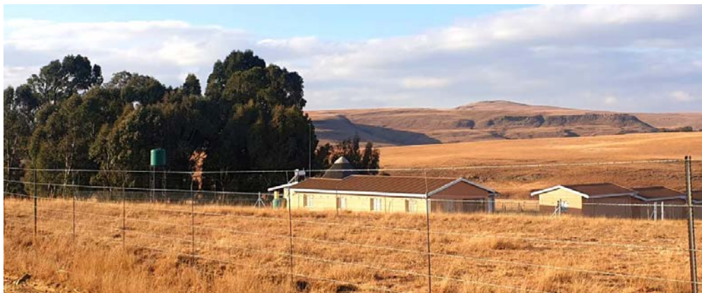
Typical example of structures to be built as part of relocation programme.
