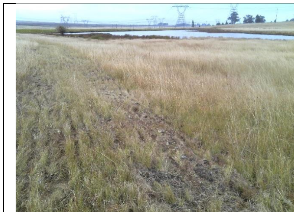
A: The dam on the southern side of the site, looking downstream
