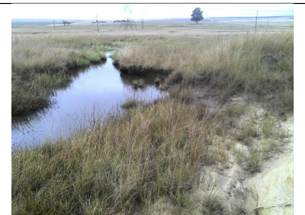
B: The spillway at the South-western end of the wall
