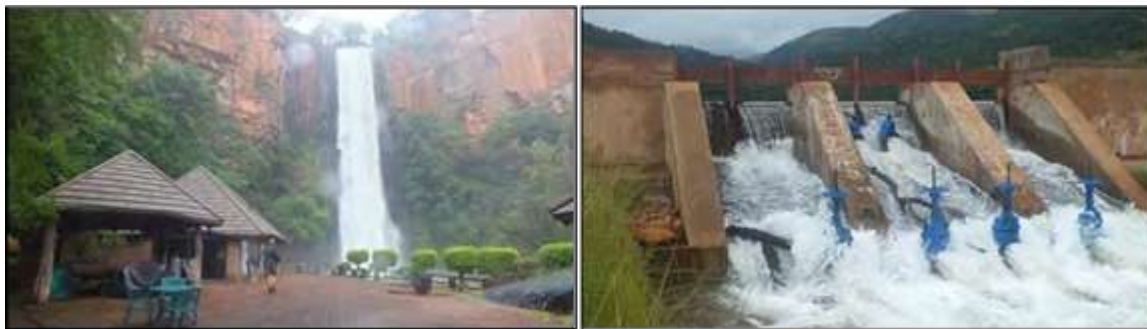
Figure 4.4.3. Fish Migration Barriers in Devil's Creek: Waterfall (A), and Existing Dam (B).
