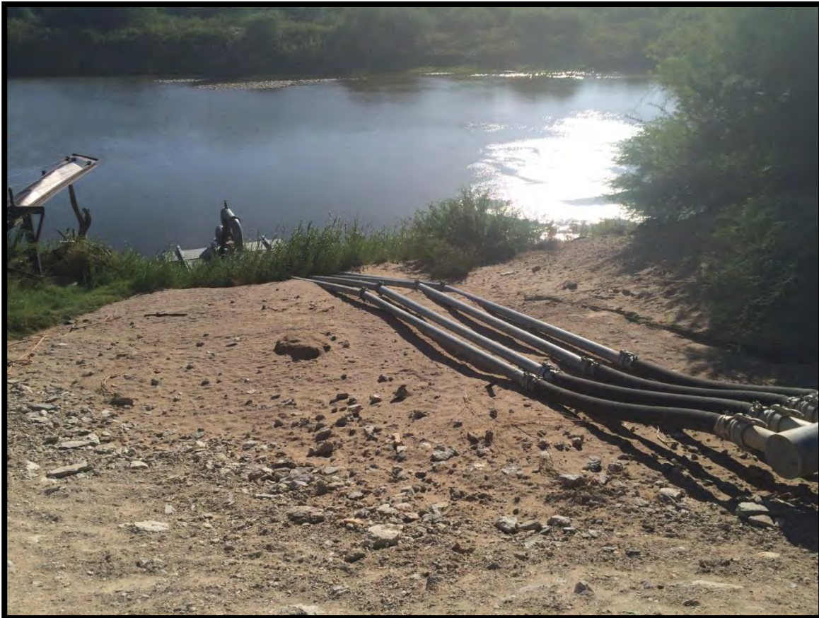
Figure 3.1: Existing water abstraction point.
