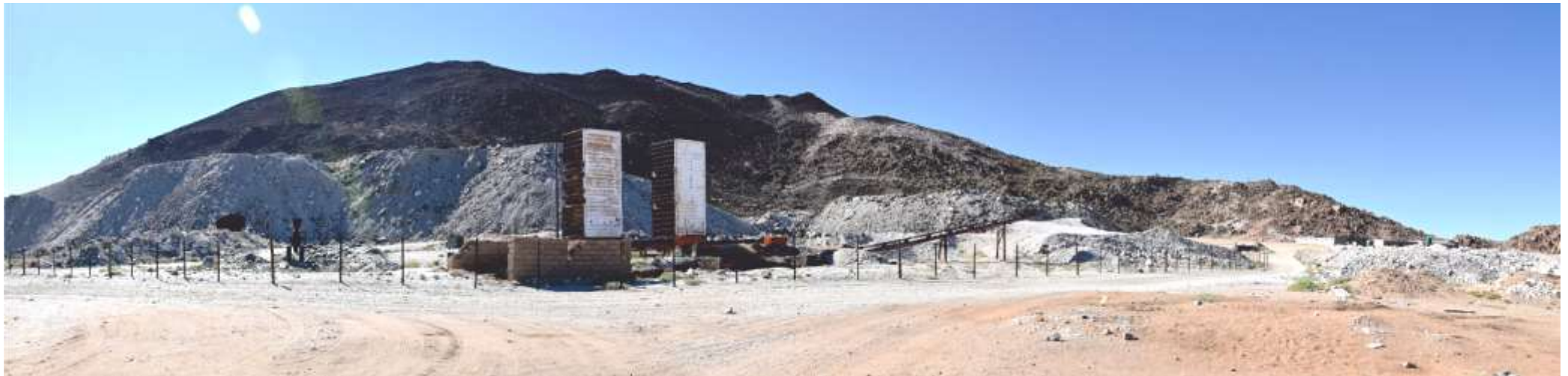
Photo 6: Remnants of the old Processing Plant with the plant residue dump in the background being reprocessed from the east.
