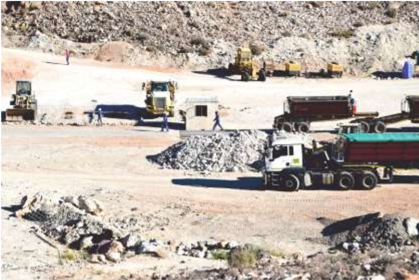
Photo 8: Weighbridge and dispatch facility
