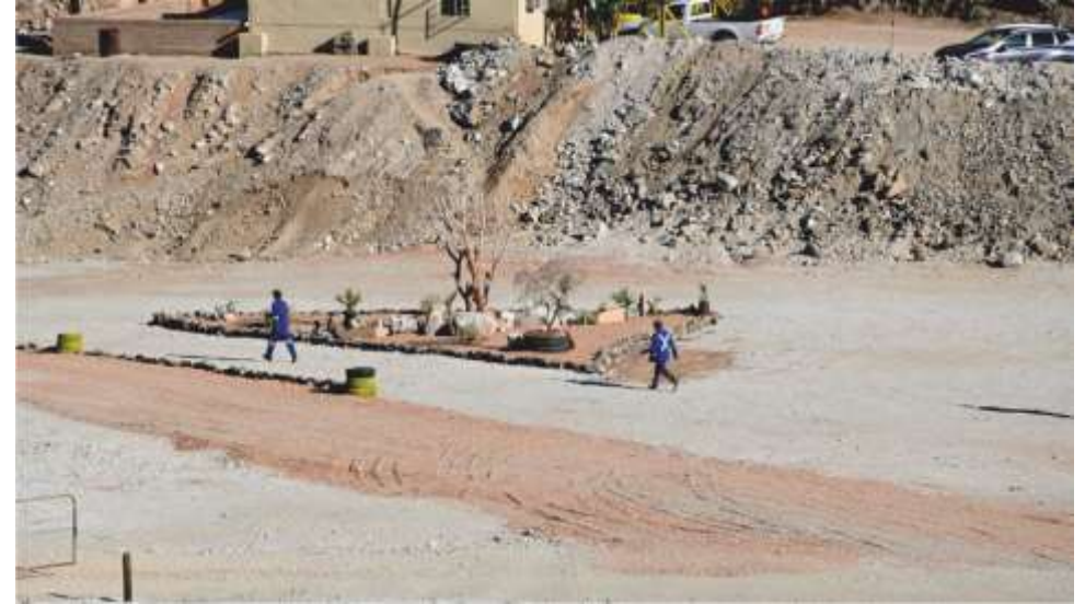
Photo 19: Recent management interventions have been initiated to improve general site condition with good demarcation of activity areas.
