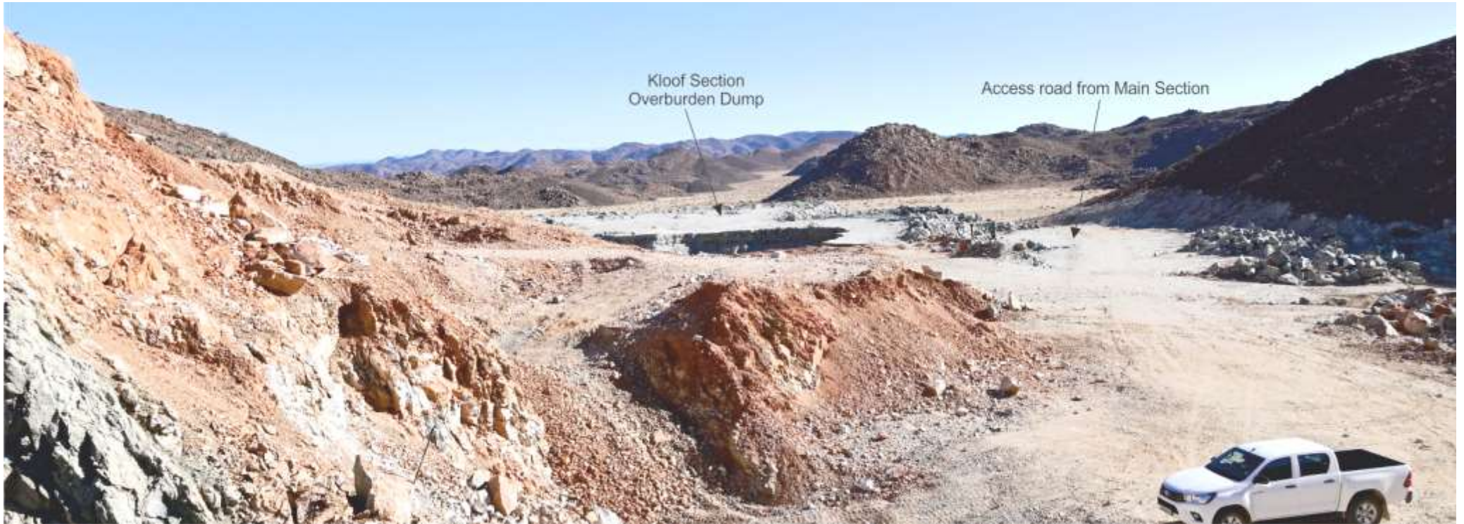
Photo 5: Looking north from the adit of the Kloof Section excavation at the main section access road and the existing waste dump.
