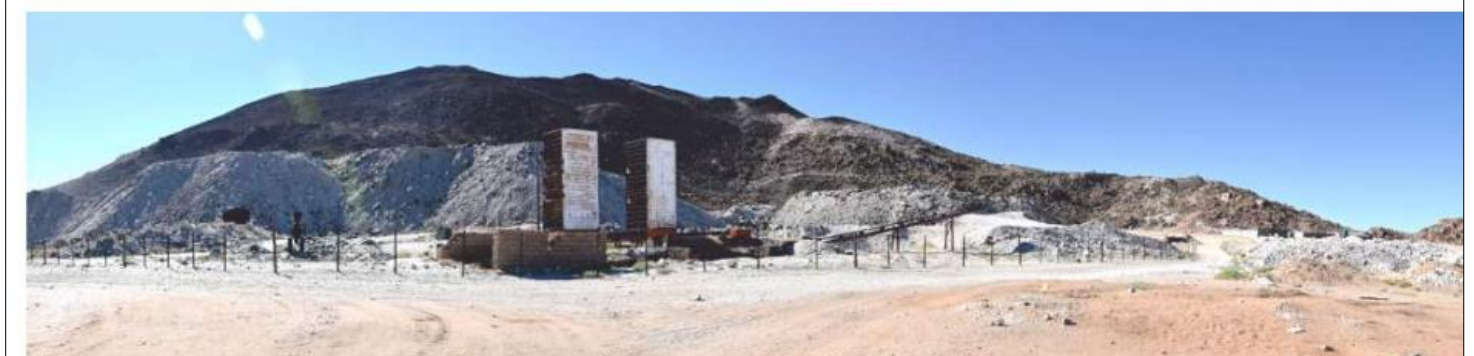
Photo 6: Remnants of the old Processing Plant with the plant residue dump in the background being reprocessed from the east.
