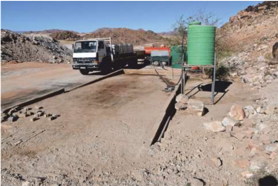
Photo 16: Wash bay facility with a very basic oil trap. Oil trap must be upgraded and covered despite very low rainfall
