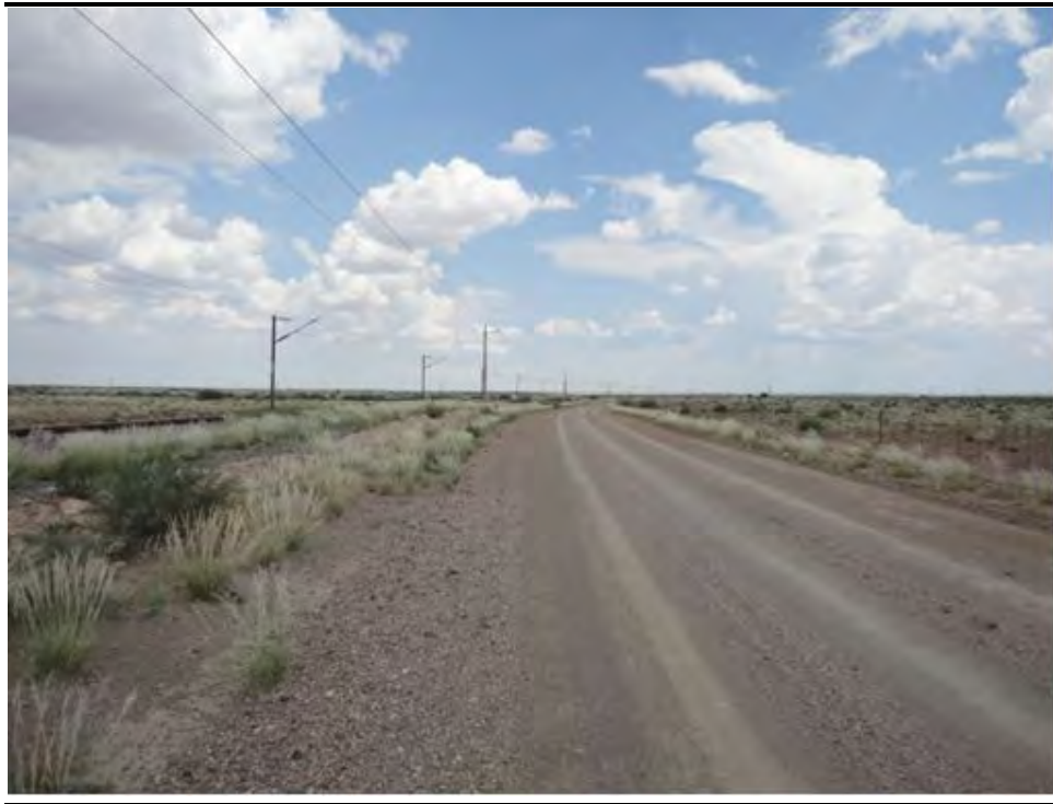
Figure 1.5 View of Sishen- Saldanha Railway Line and Service Road
