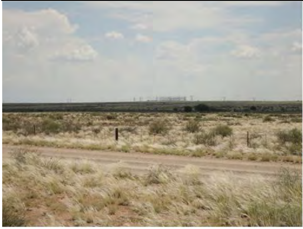
Figure 1.3 Typical Vegetation of the Site with Eskom's Aries Substation and Power Lines
