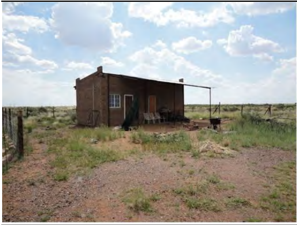
Figure 1.11 Existing Labourers Cottage on Olyven Kolk Site
