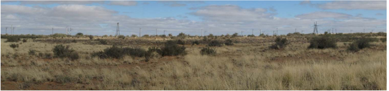
Panoramic view south to south east showing existing vertical nature of the power line modifications to the landscape (GPS 024, Plate 25:GPS Point Map)
