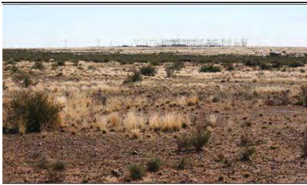
Figure 4.3 Aries Substation in background
