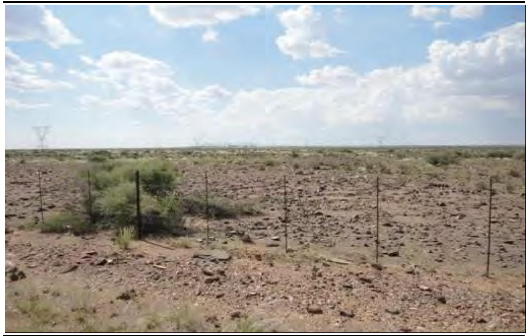
Figure 6.12 Eskom's Aries Substation in the Distance
