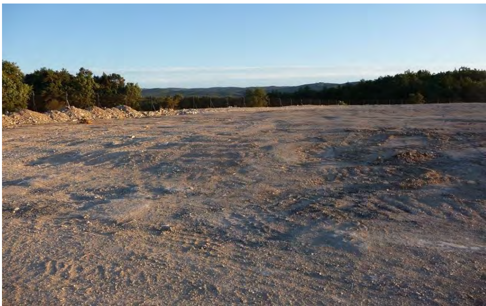
Figure 2: Example of site clearing (Source: ERM)
