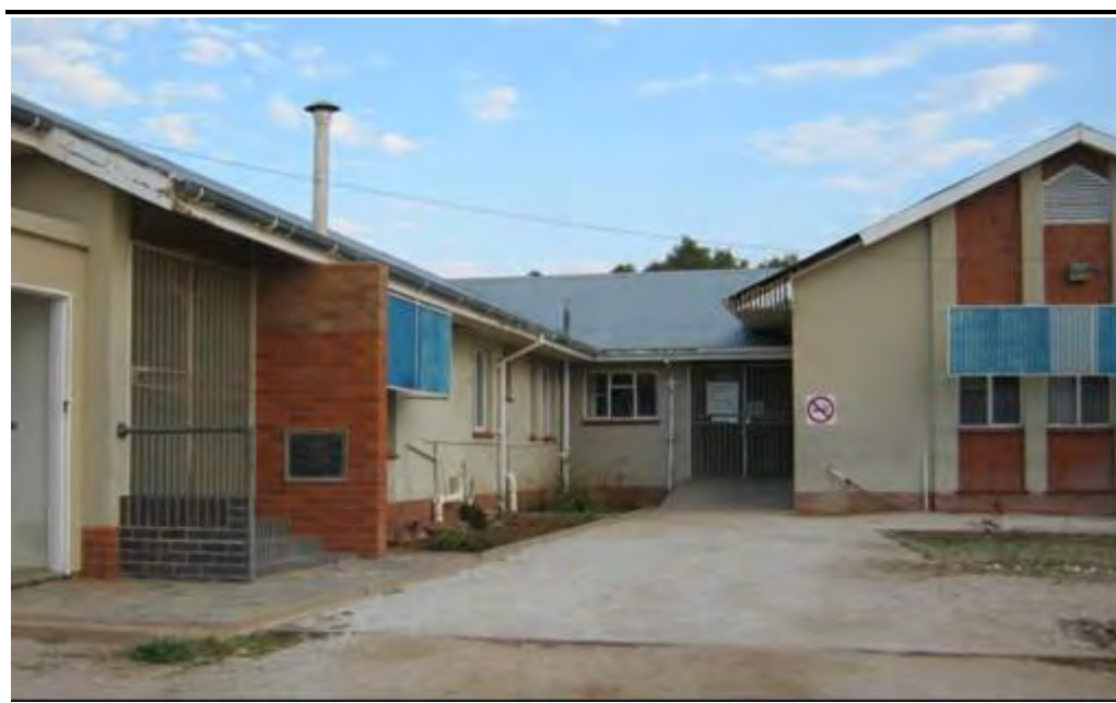
Figure 6.6 Kenhardt Community Health Centre (CHC)
