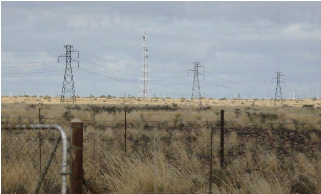
Figure 2: Existing industrial infrastructure (GPS 14)
