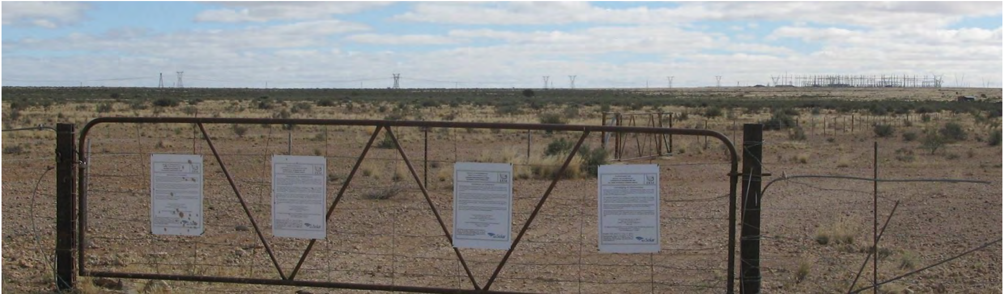
Figure 1: Existing site entrance gate looking towards Aeries sub-station (GPS 023)
