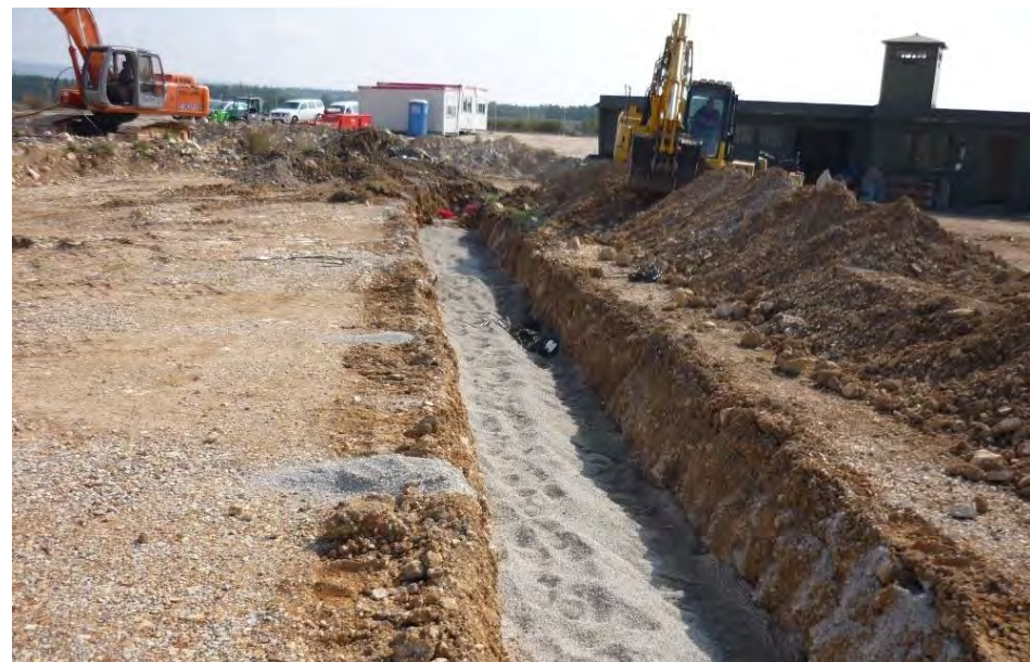
Figure 3: Example trench construction (Source: ERM)
