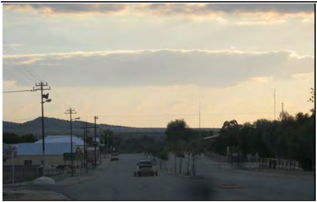
Figure 6.16 Tarred Main Road (R27), Kenhardt
