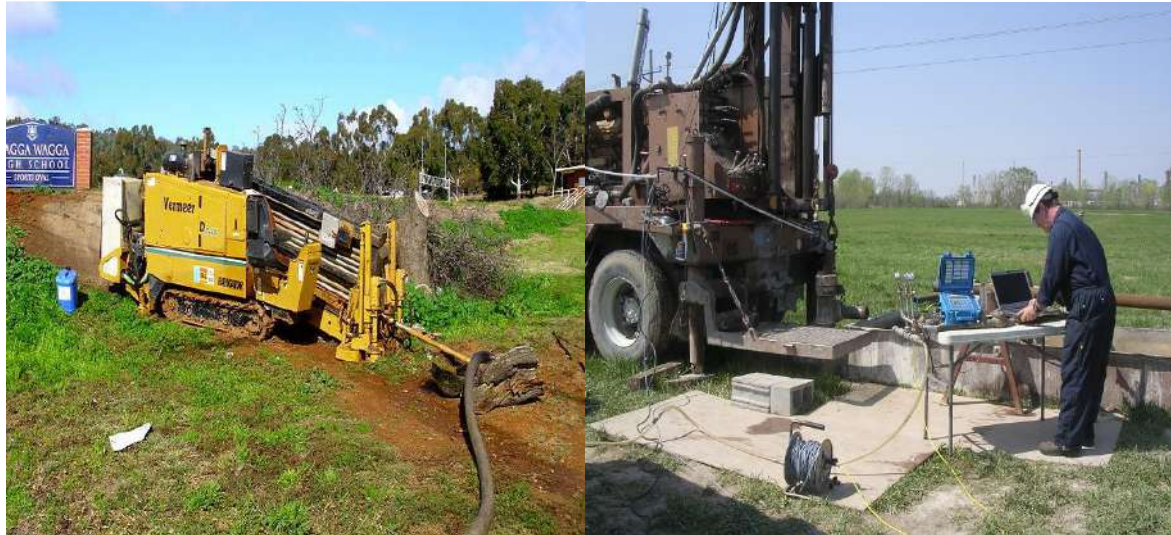
Figure 10: Directional drilling and Geophysical down-hole survey
