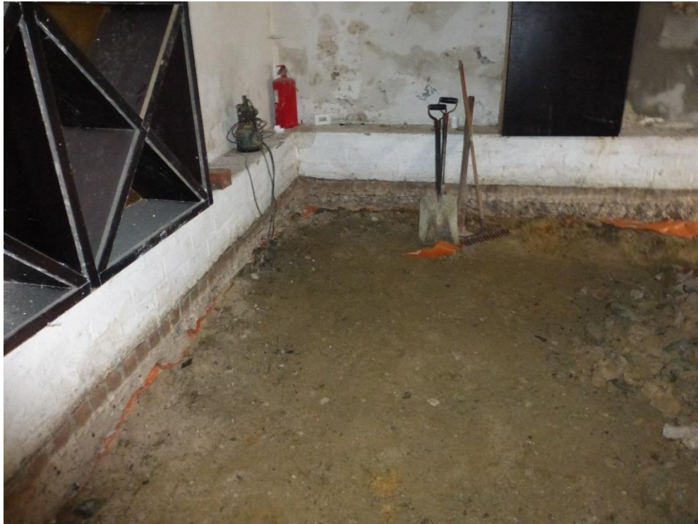
South western corner of the cellar excavated down to the previously excavated level. The base layer is predominately clay with some small rocks.
