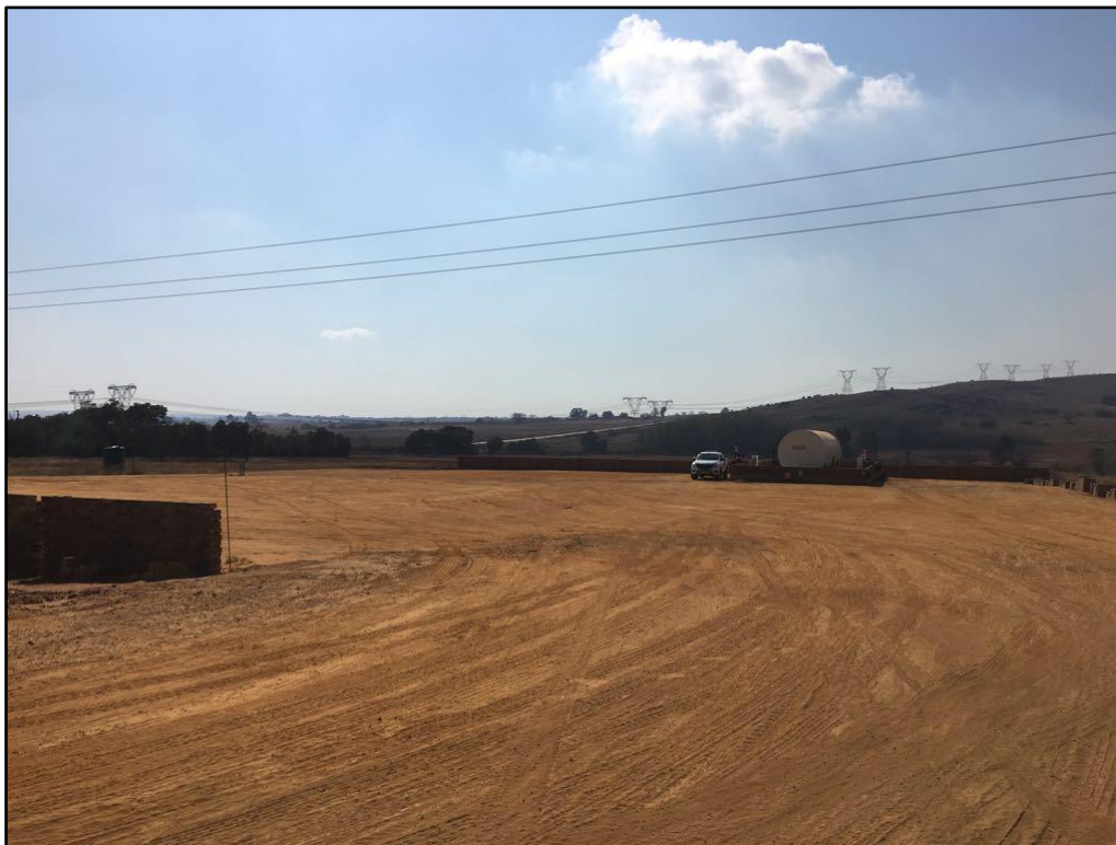
Figure 1: Current status of the development site (17 August 2016)
