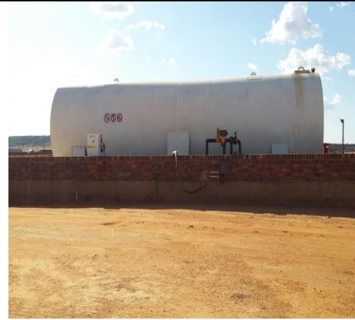
Figure 9: South - Existing fuel depo with a diesel tank.
