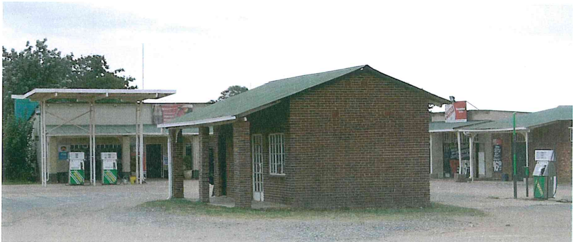
Figure 2-2: Kleinsonderhout Filling Station
