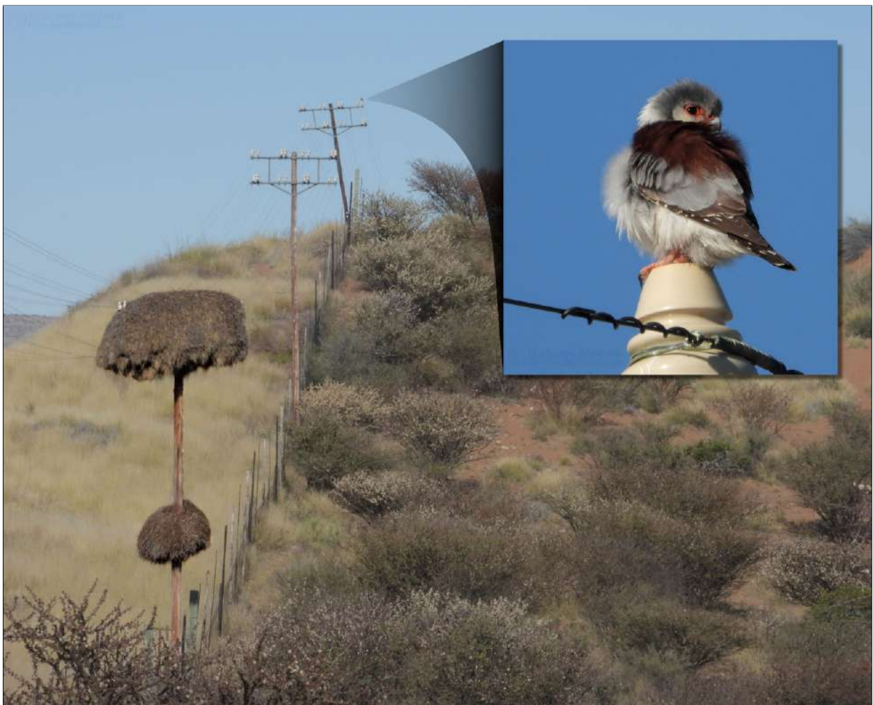
Figure 41: Examples of the utilisation of pole and wire infrastructure by birds in the immediate vicinity of the ORSF1 power line.
