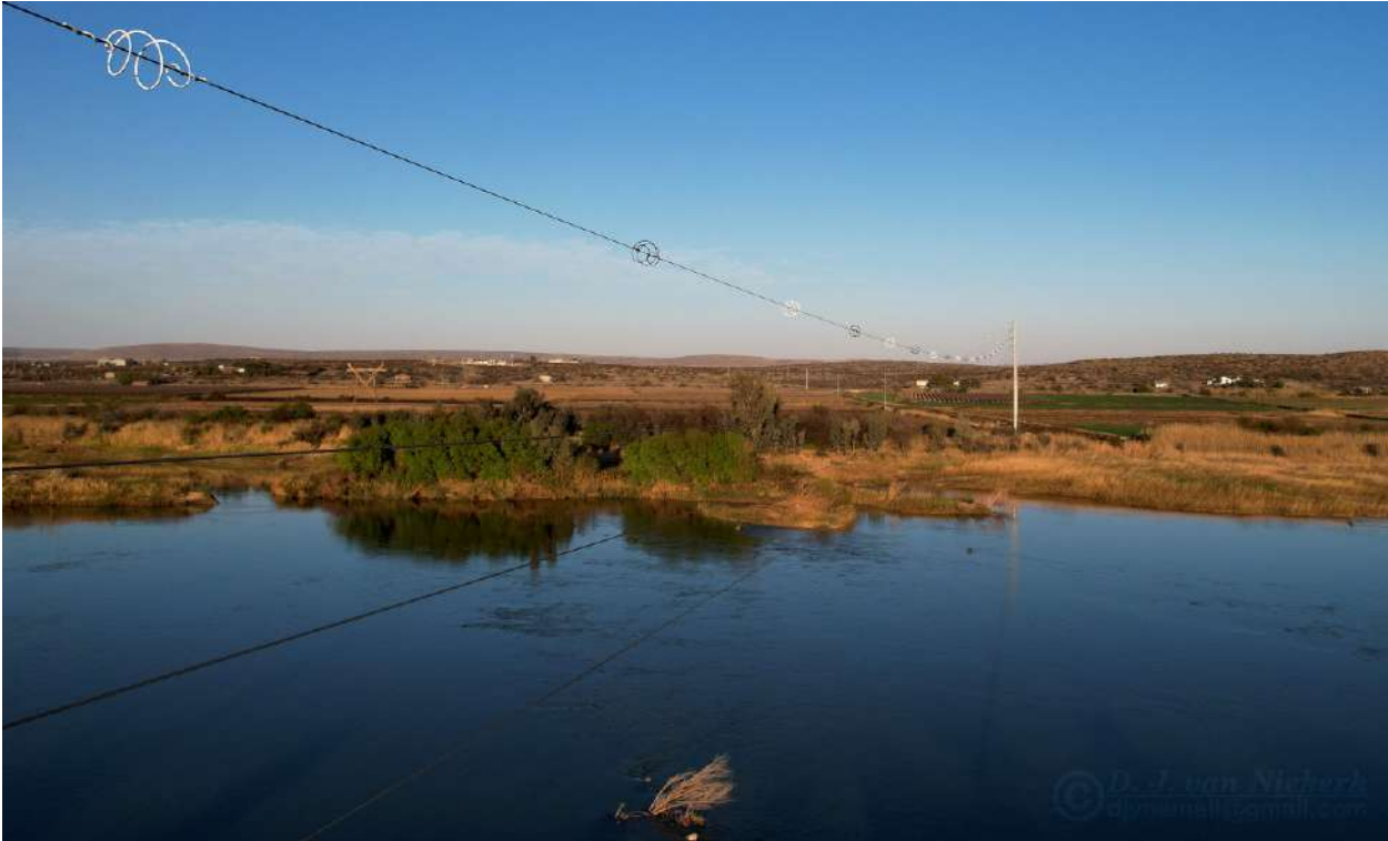
Figure 53: The proposed spacing of markers on the ORSF1 power line. See Section 7.4 (page 84).
