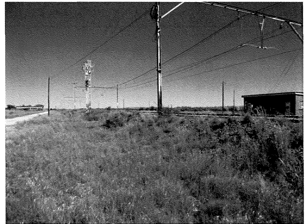
The area is already disturbed due to the rail line.
