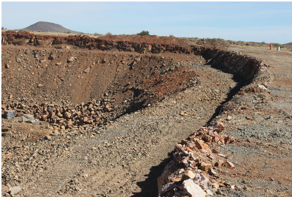
Photo 4: Example of upper perimeter safety bench before perimeter shaping and fencing on another site planned by SPC
