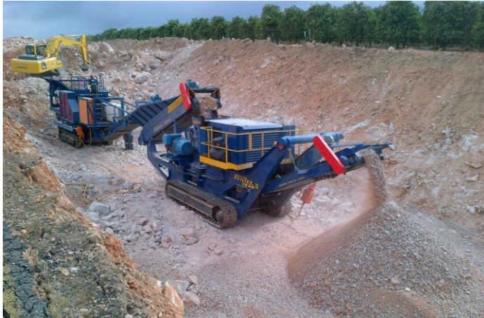
Photo 3: Typical mobile tracked in-pit crusher on another contract by the Applicant
