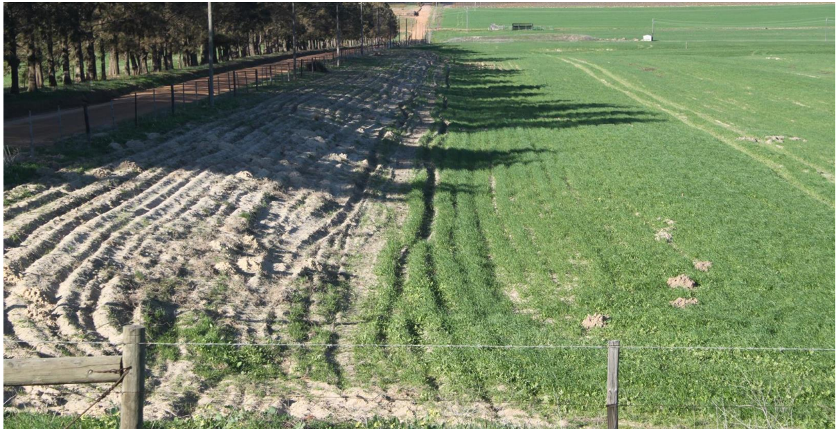
Photo 13: Typical Borrow Pit rehabilitation in process, with full topsoil replacement and revegetation by pasture seeding on the floor of the excavation, and scarification of 1:3 side slope ready for hand seeding.
