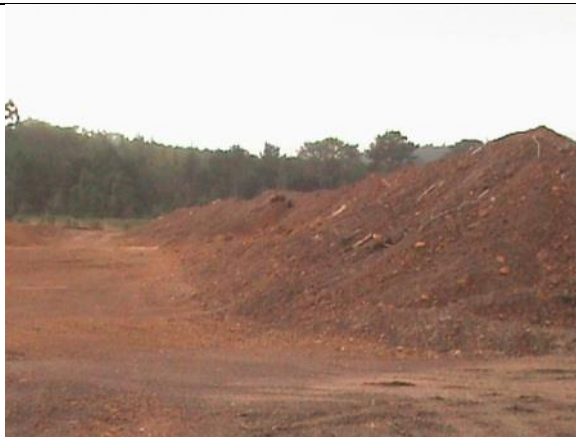
Photo 4: Example of temporary perimeter topsoil stockpiles (berms)
