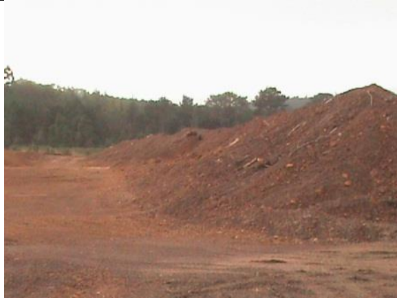
Photo 4: Example of temporary perimeter topsoil stockpiles (berms)
