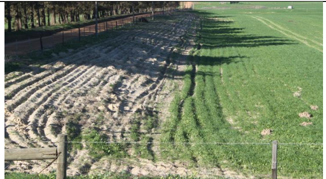
Photo 7: Example of perimeter sloping to 1:3 following retopsoiling and revegetation of a typical wedge-shaped excavation in "soft" materials
