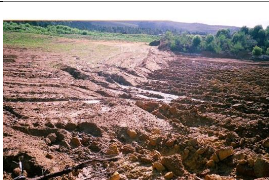
Photo 6: Example of growing medium/topsoil replacement in a gravel pit
