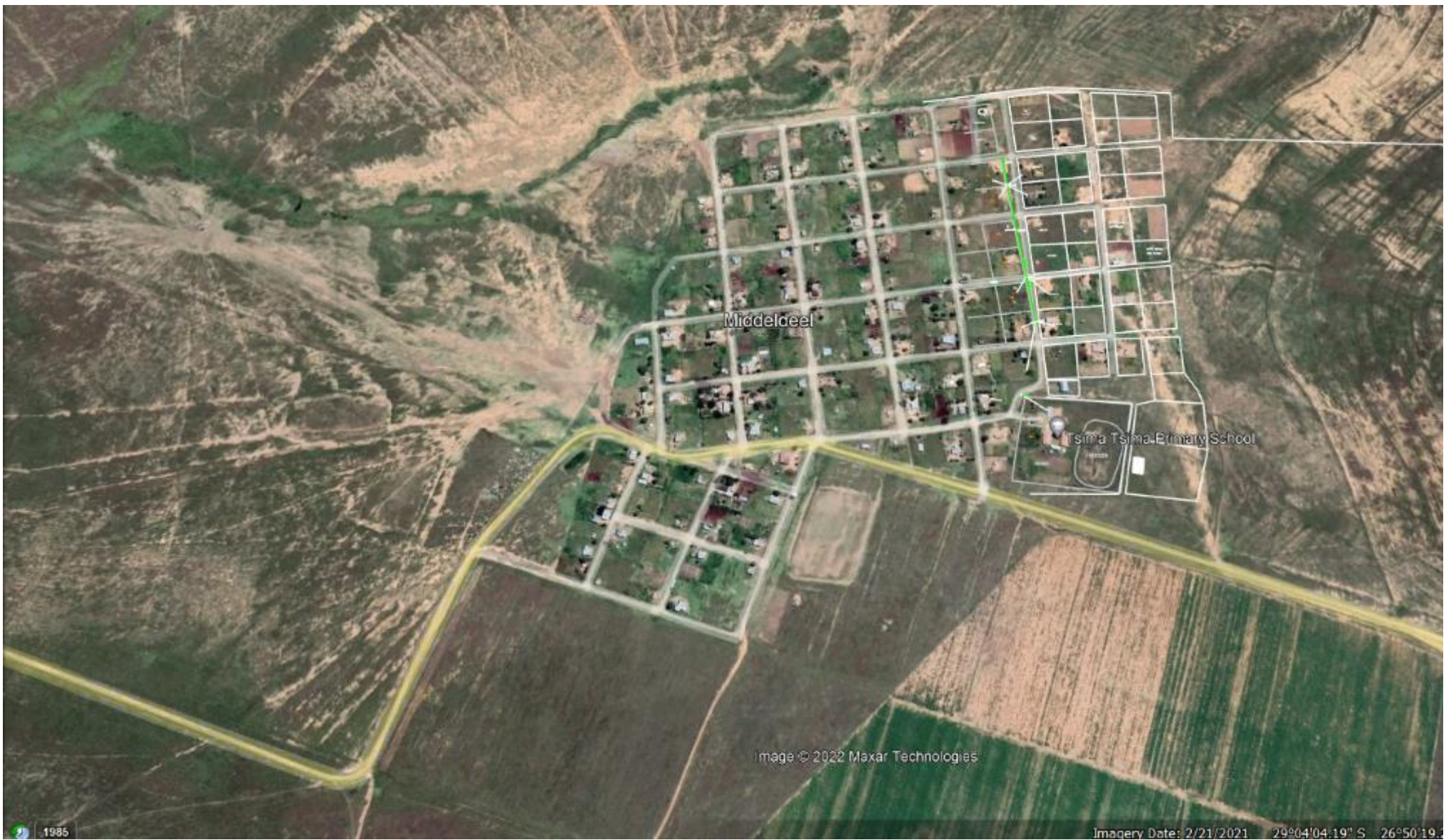
FIGURE 10: MIDDELDEEL VILLAGE WITH ALLOCATED NEW STANDS TO BE ELECTRIFIED
