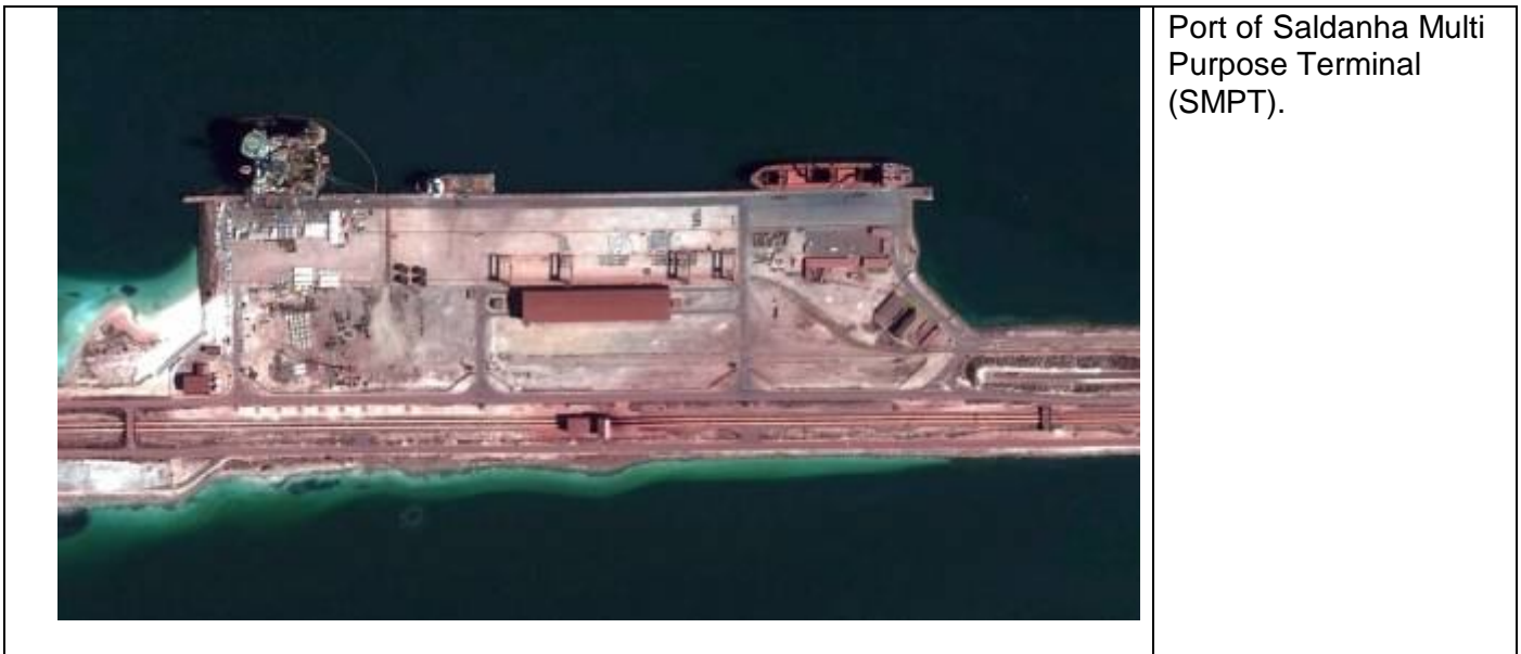
Overview of the Port of Saldanha Multi Purpose Terminal (SMPT)
