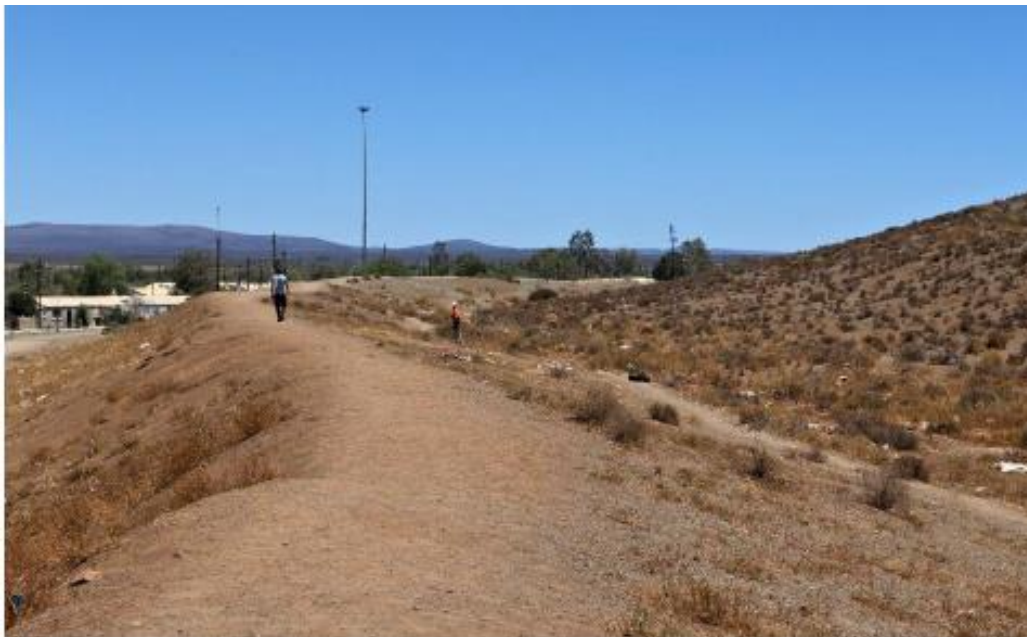
Figure 3: Large berm constructed to the north of the town to divert runoff from the slopes of the Hantam Mountains towards the trench and around the urban area, as part of stormwater management.
