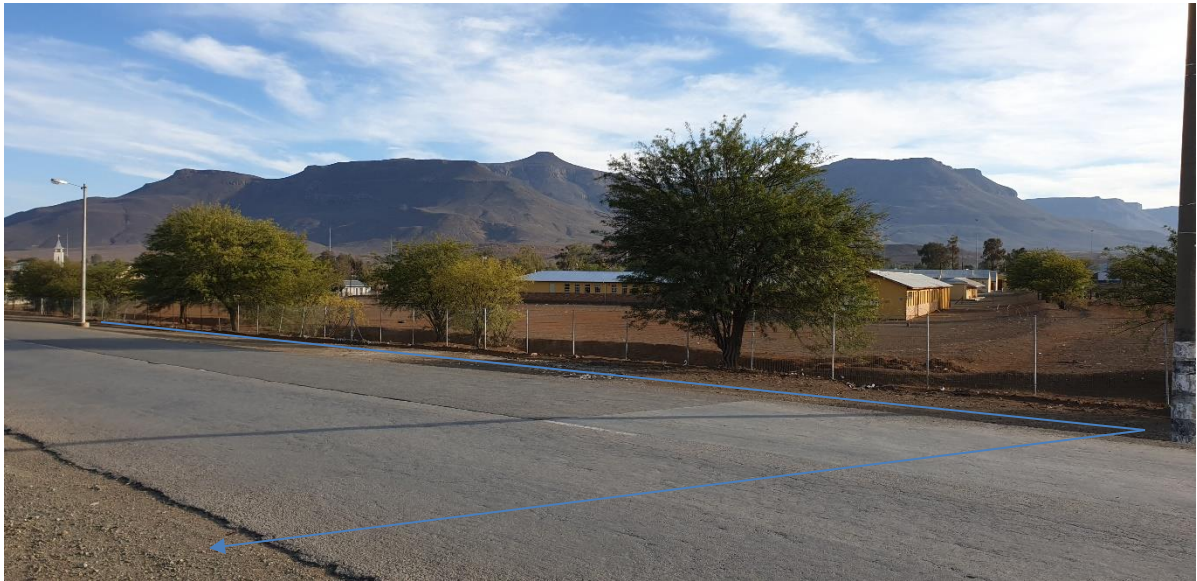
Figure 13: Pipeline route to run parallel with the fence next to the school from where it is proposed to cross the R355, Point H on Locality maps.
