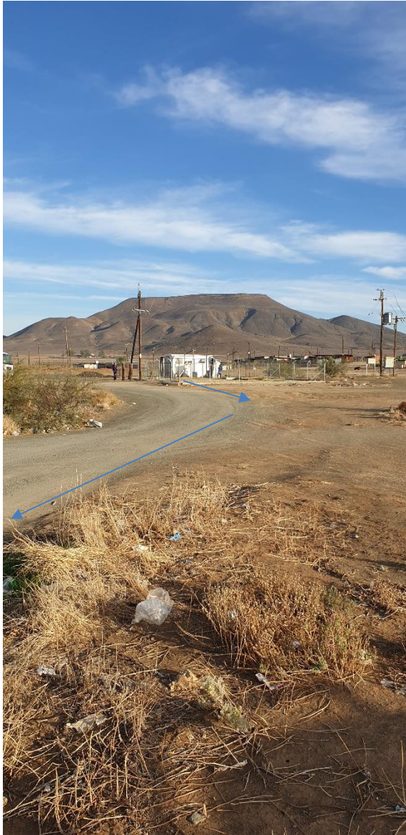
Figure 5: Existing pump station in the background from where proposed pipeline is to start
