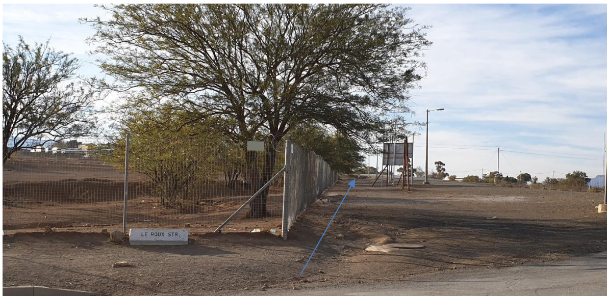
Figure 13: Pipeline to cross Le Roux street, point G on the locality maps, and run parallel to the fence next to the school towards Hantam Park Showgrounds.
