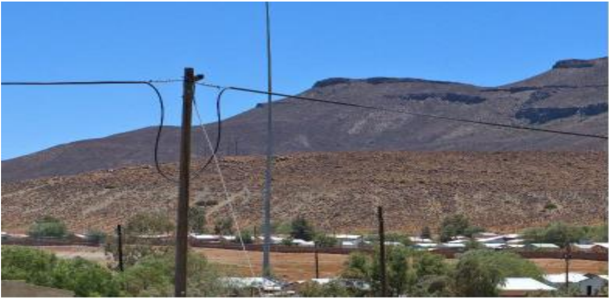
Figure 9: De Kraal Sport Grounds, pipeline to terminate in n 120KL reservoir. Point H in locality maps.
