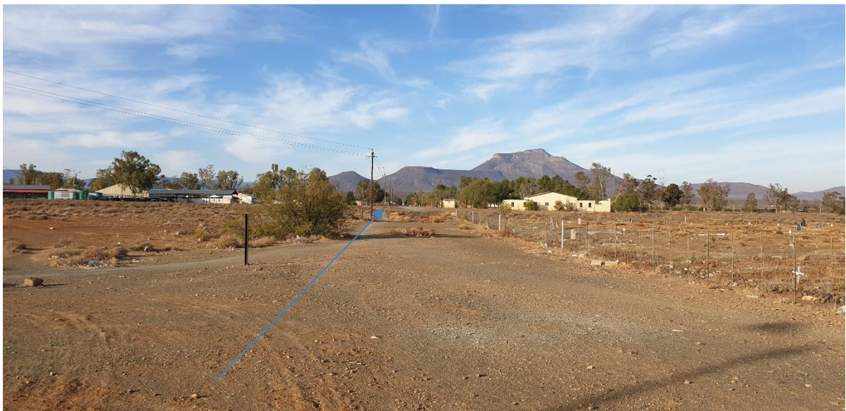
Figure 14: Pipeline route to fall on the gravel road next to the cemetery towards the Hantam Park Showgrounds. Approximately point I on locality maps.
