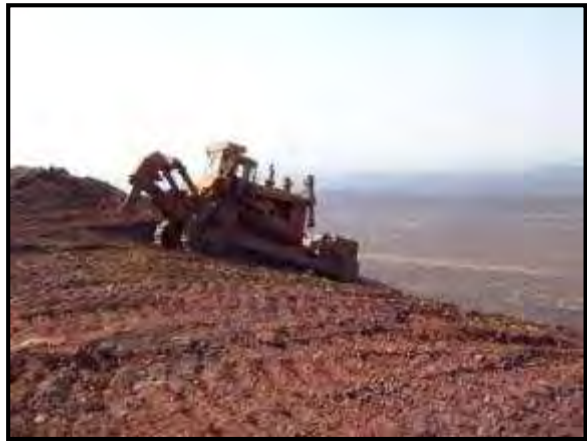
Mechanically reducing angle of slop
