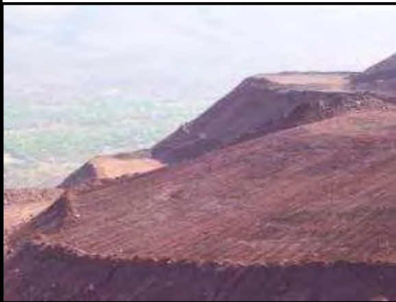
Slope reduced to a 20° angle
