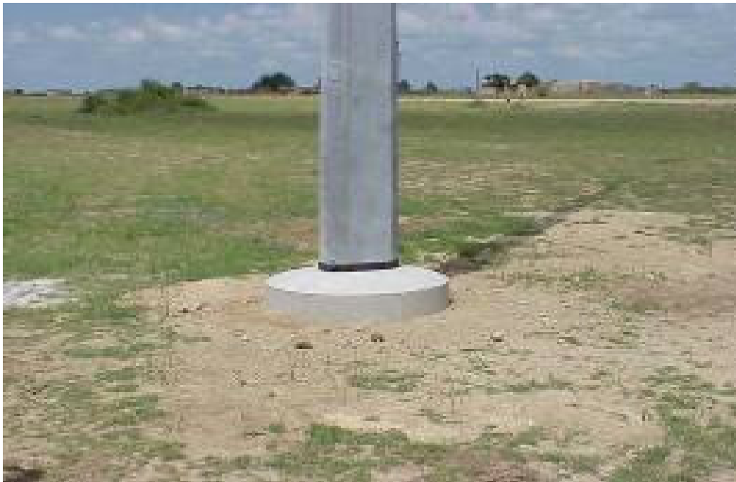
FIGURE 2: PYLON EXCAVATION FOUNDATION (SOURCE ESKOM)
