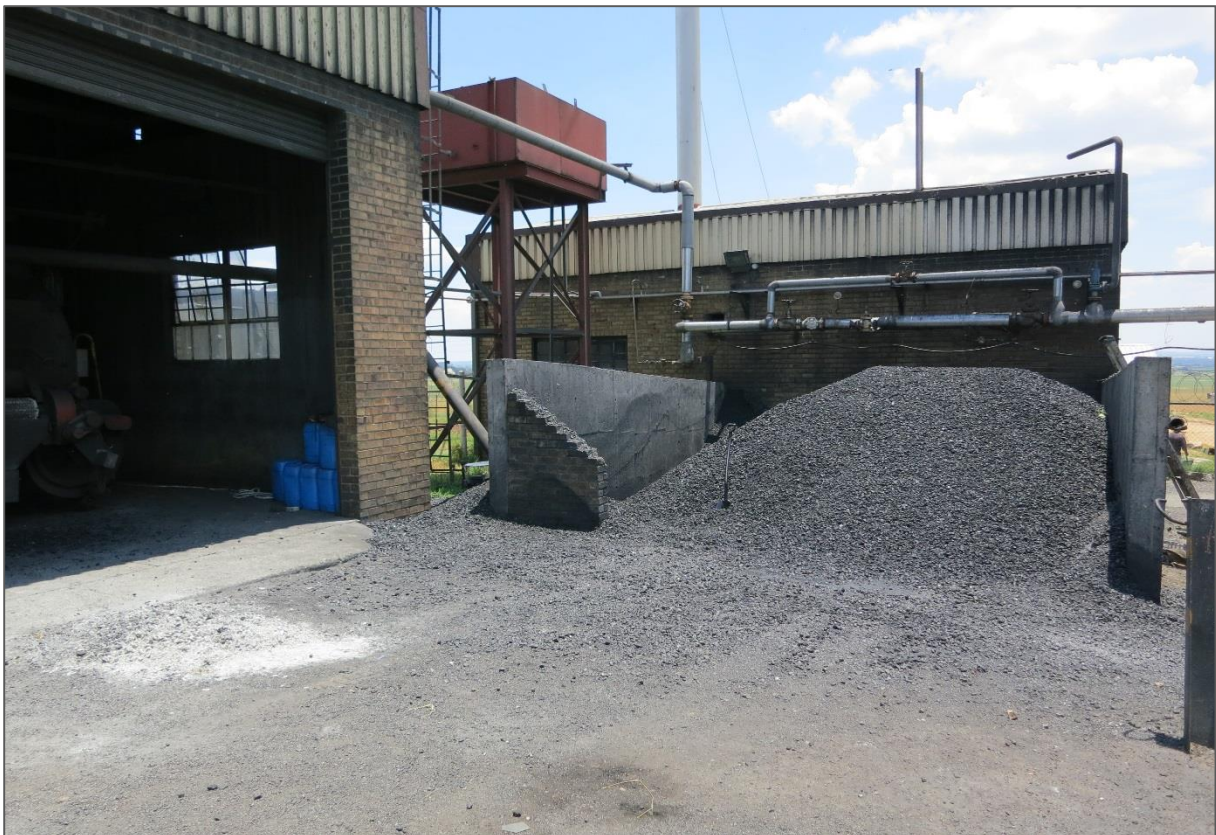
Figure 6: The coal storage bunker
