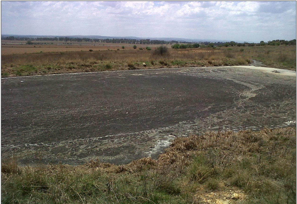
Figure 17: The existing wastewater evaporation pond
