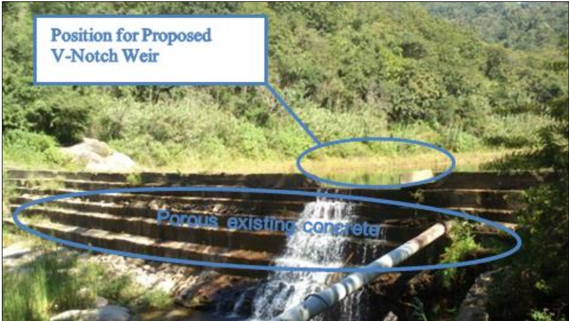
Figure 3: Position for the Proposed V-Notch Weir
